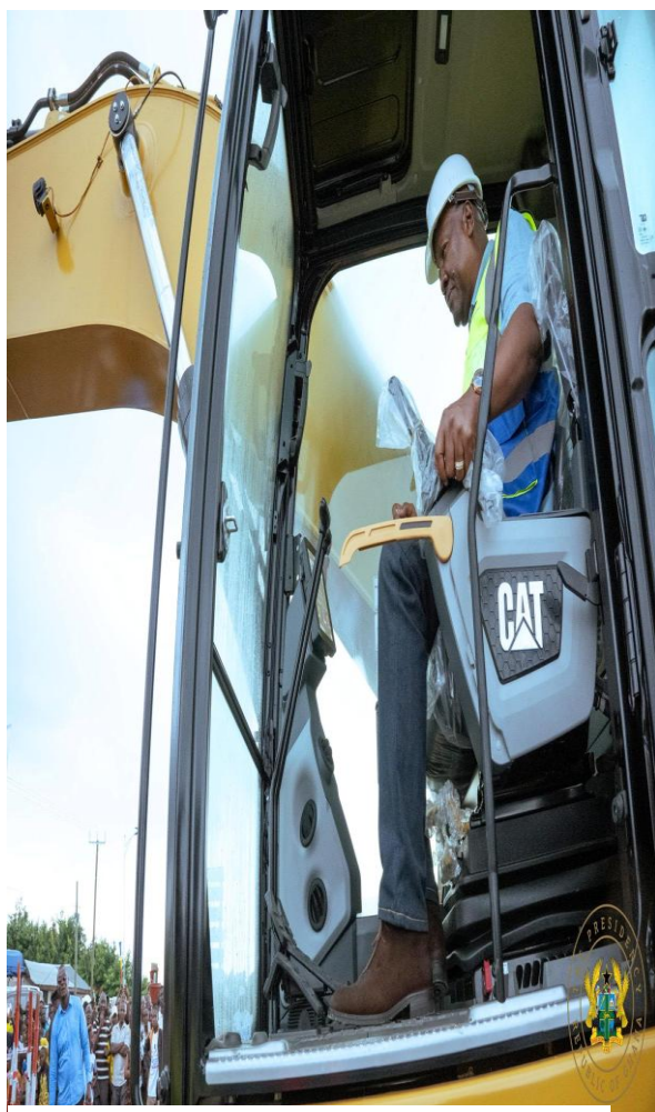
Sodcutting of Dodowa-Afienya Road
