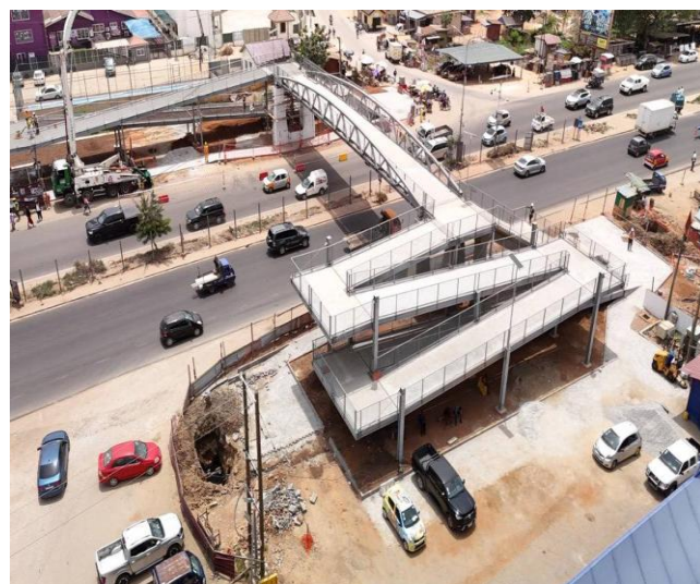
Tetegu Pedestrian Bridge
