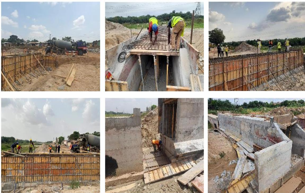
Construction of Box Culvert at Km11+613
