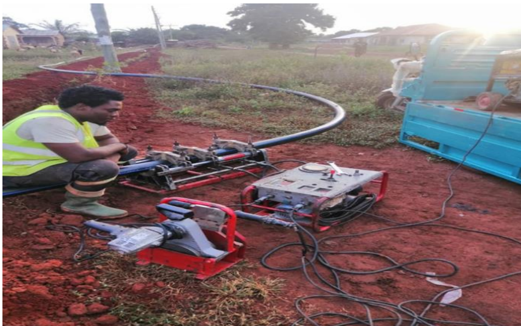
Butt welding ongoing
