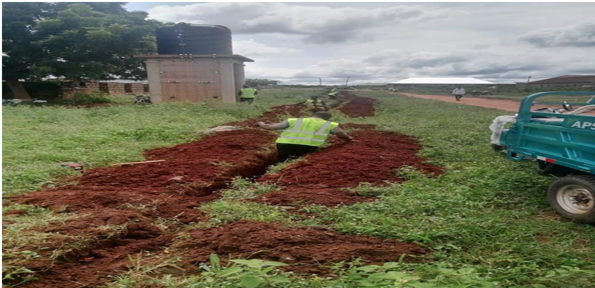
Trenching for pipe laying at Ejura
