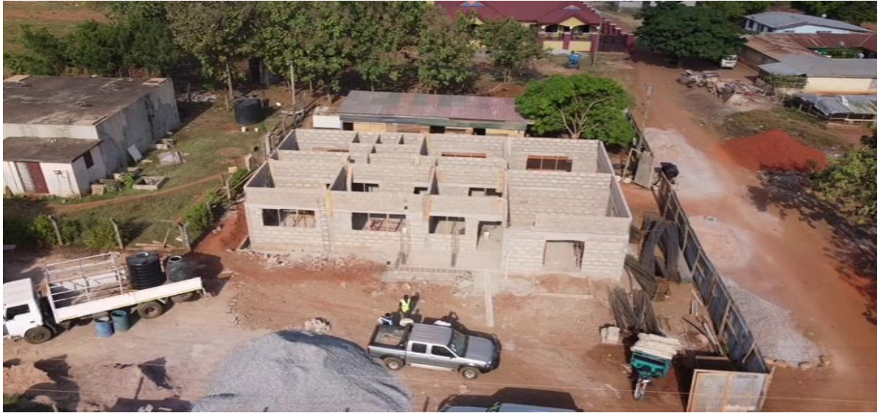
On-going construction of CWSA Office at Ejura
