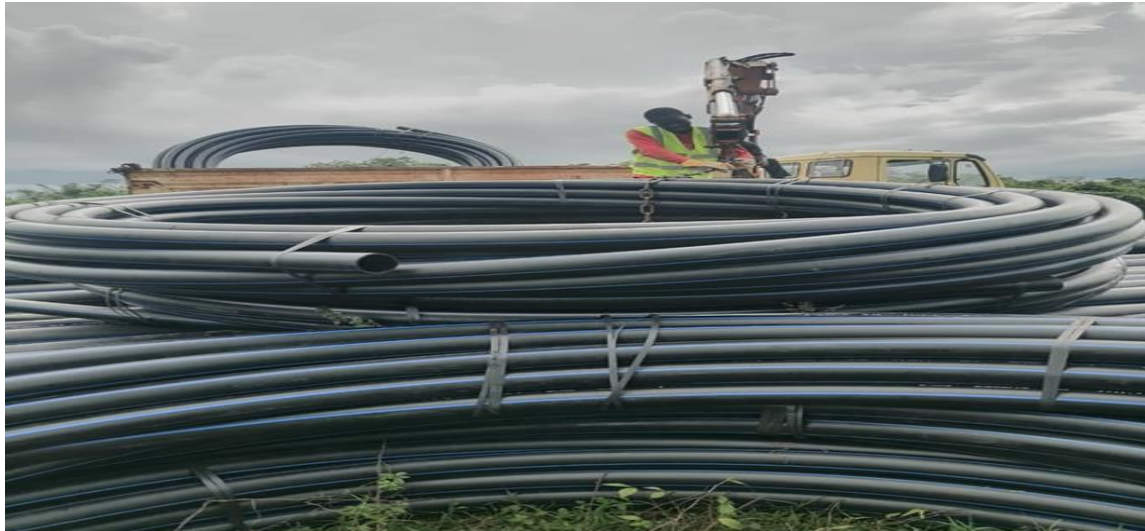
Pipe materials on site
