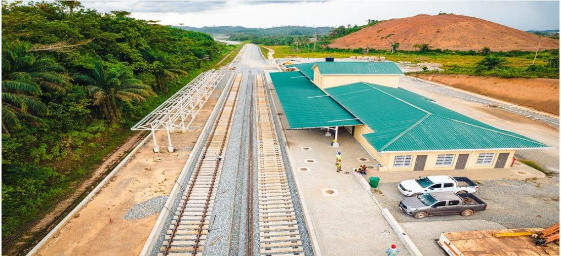
Manso Railway Station (chainage 28+633) – 92% complete
