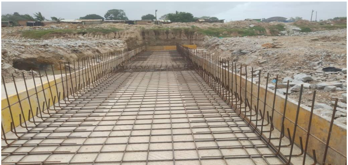
Construction of Culvert at Kaase
