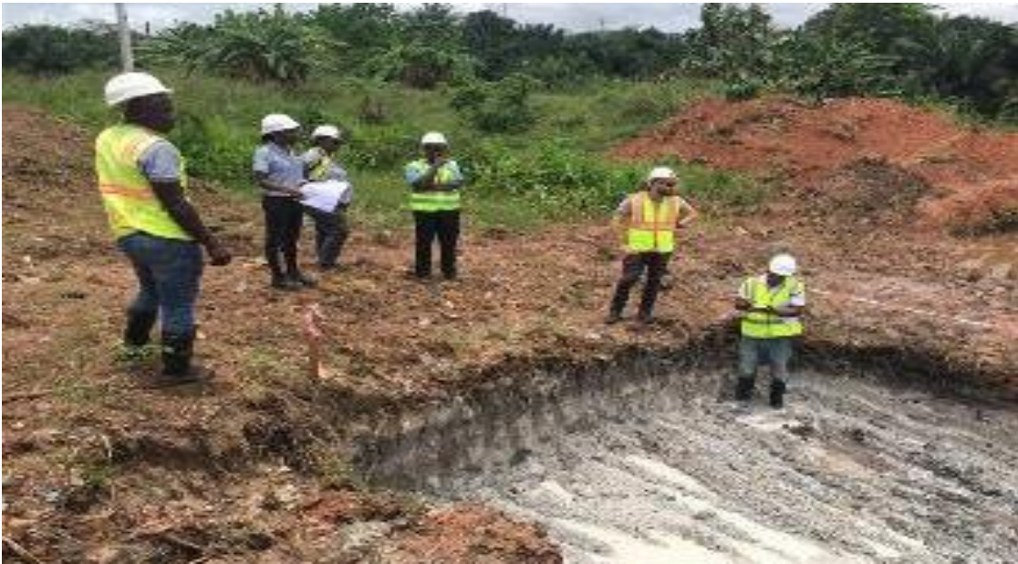
On-going Earthworks at Kaase
