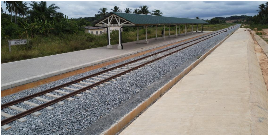
Angu Halt (chainage 21+663) – 90% complete
