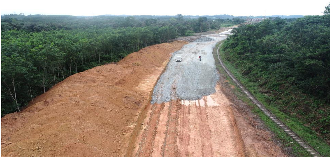
Soil Replacement Works at chainage 70+600, Tarkwa
