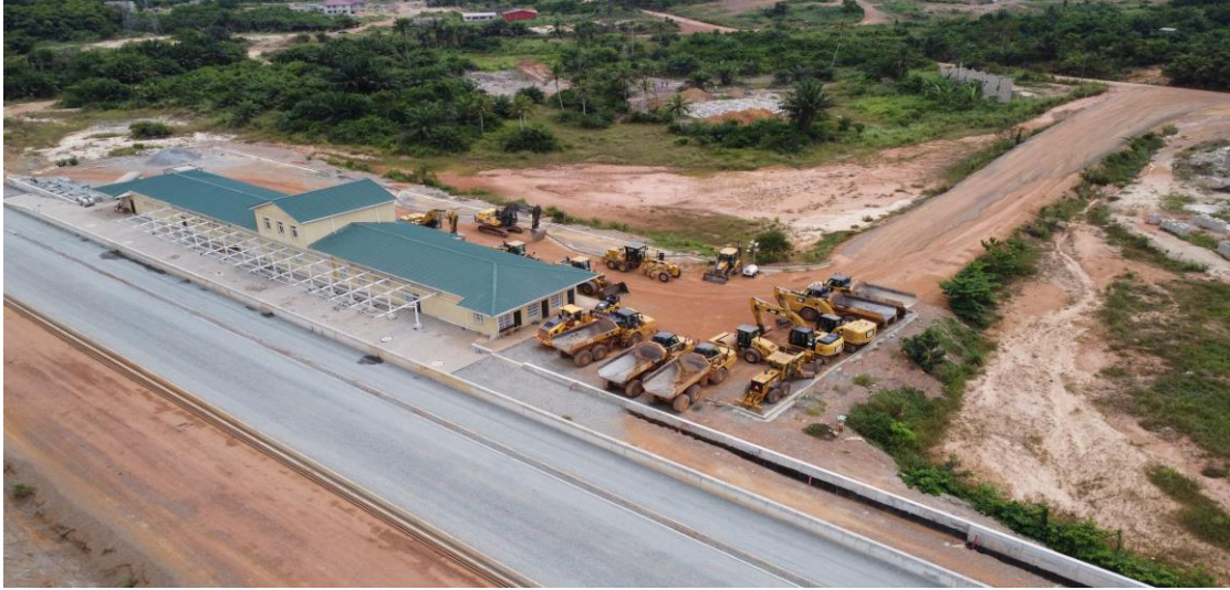
Eshiem Railway Station (chainage 15+640) – 85% complete
