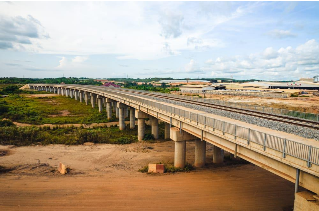
Eshiem Viaduct on the Kojokrom-Manso Railway Line
