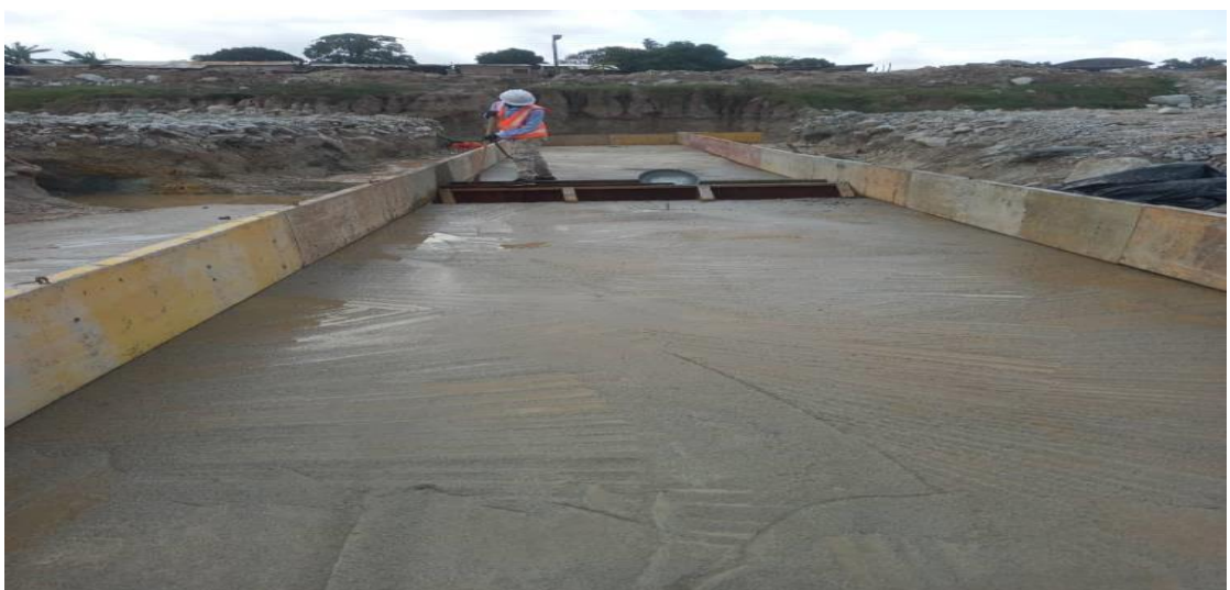
Construction of Culvert at Kaase
