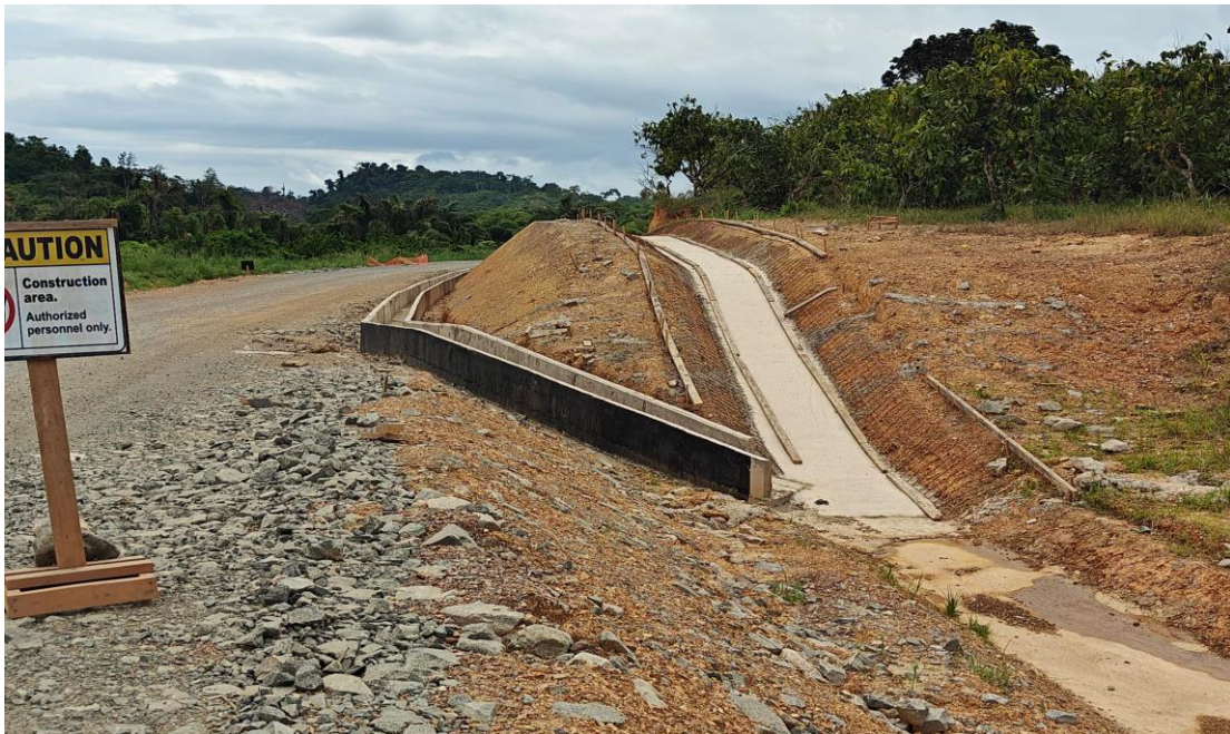
Longitudinal Drain from chainage 33+815 to chainage 33+850
