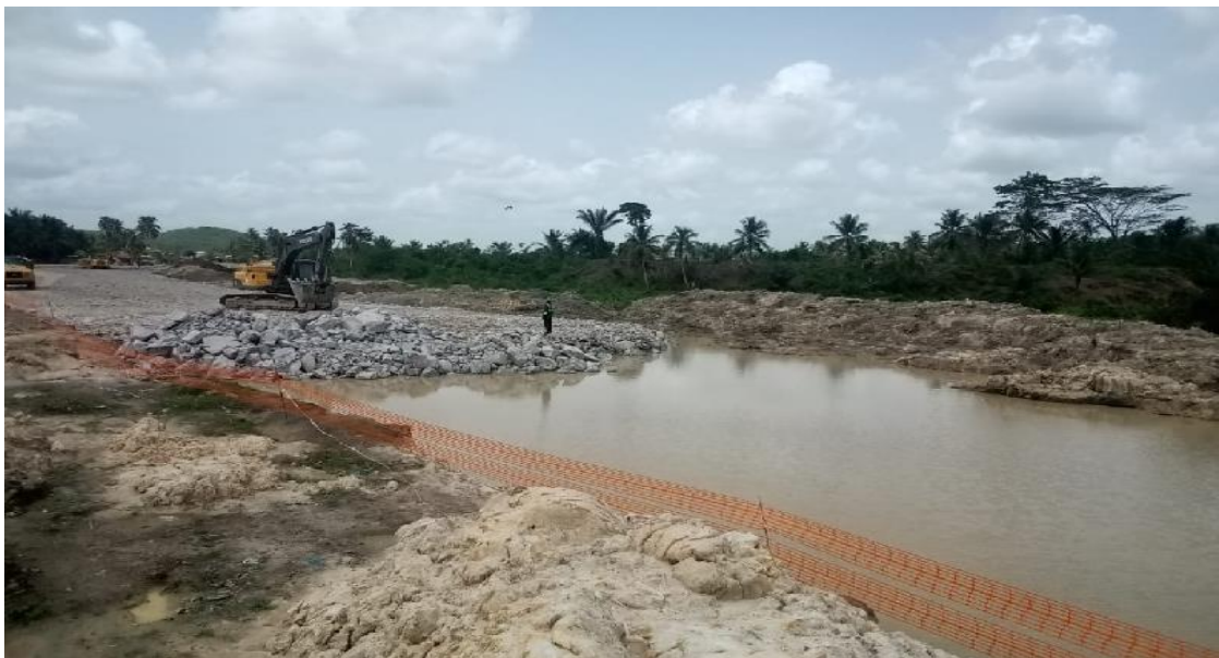
Soil Replacement Works at chainage 42+500, Benso
