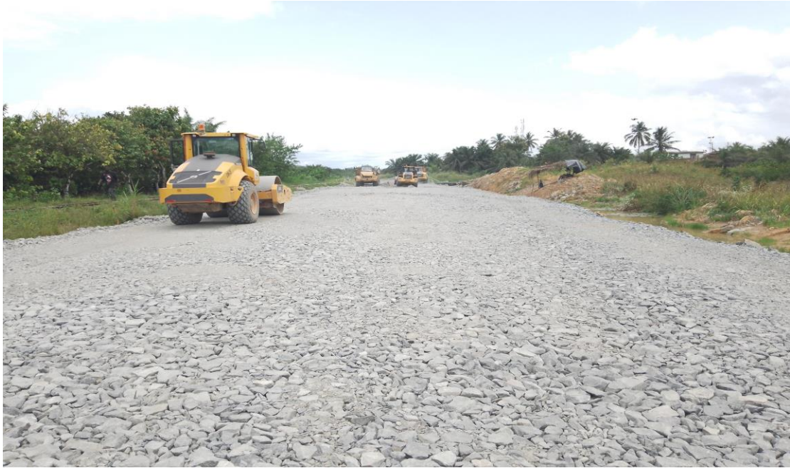
Embankment at chainage 40+859, Amantin
