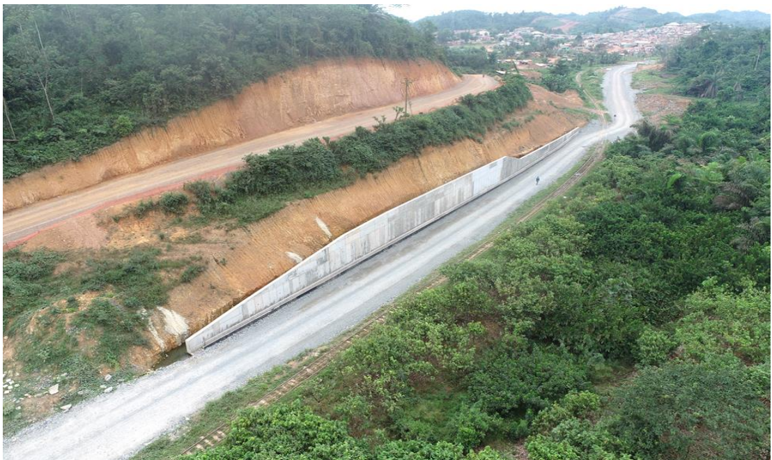
Retaining Wall at chainage 36+292, Amantin
