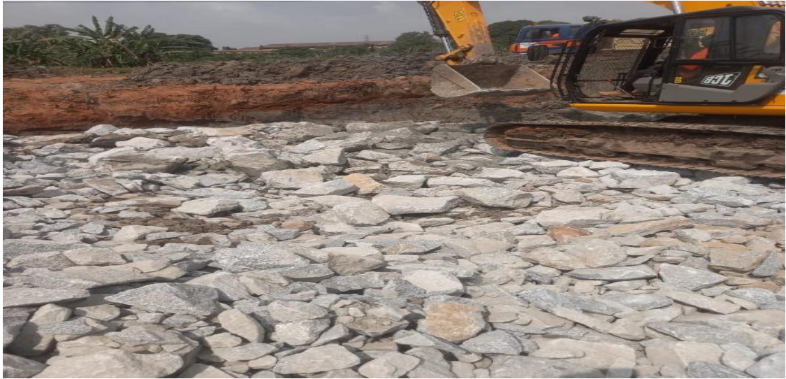
Earthworks Rock Stabilization at Kaase
