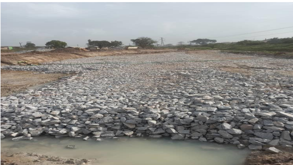
On-going Earthworks at Kaase
