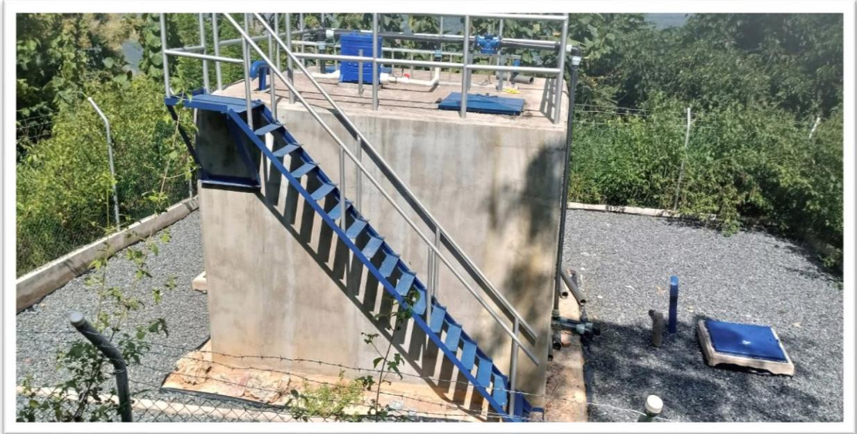
**Ground Level Concrete Storage Tank of Abutia Agorve Water Supply System in the Volta Region under the WSIP-DSDP**
