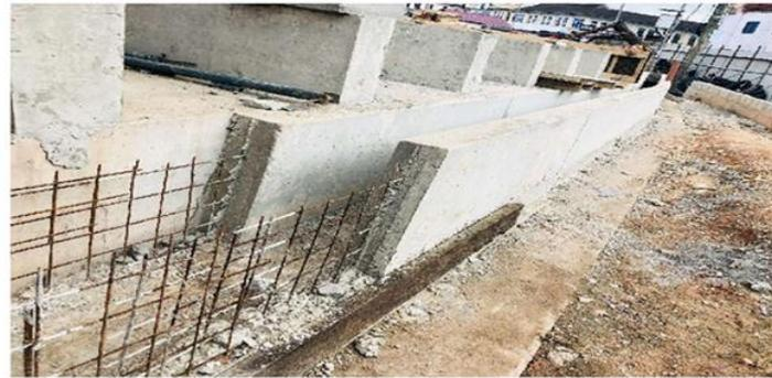
HTA 4- Concrete casting for U-drain – 23-September-22
