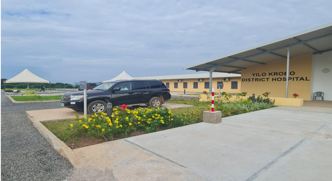
Yilo Krobo District Hospital
