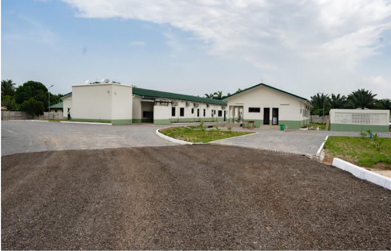
Dodowa Treatment and Holding Centre
