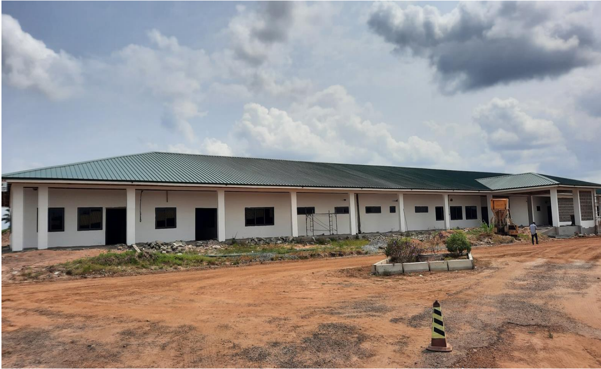
Adaklu Treatment and Holding Centre
