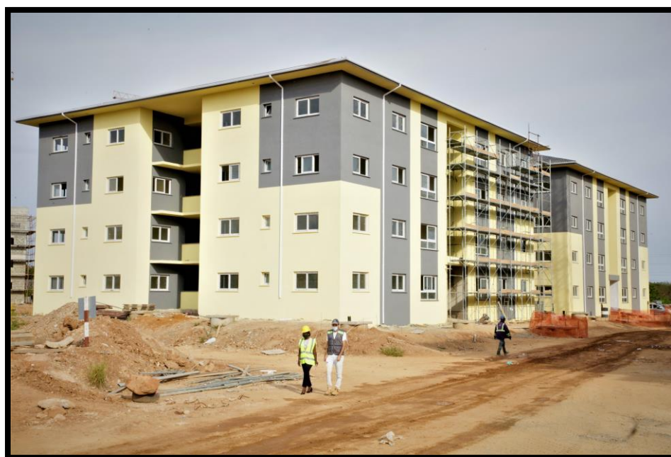
Figure 2: Security Services Hosing Project (Phase III)
