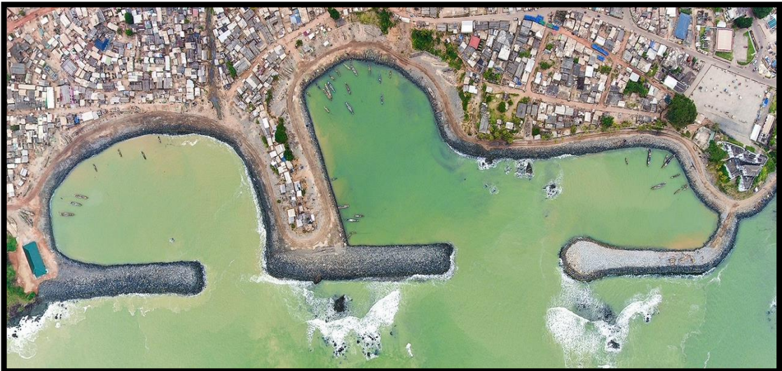
Figure 5: Axim Sea Defence Project
