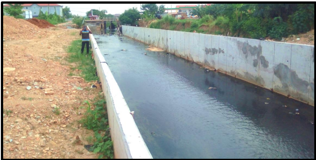
Figure 11: Haatso Drainage Project
