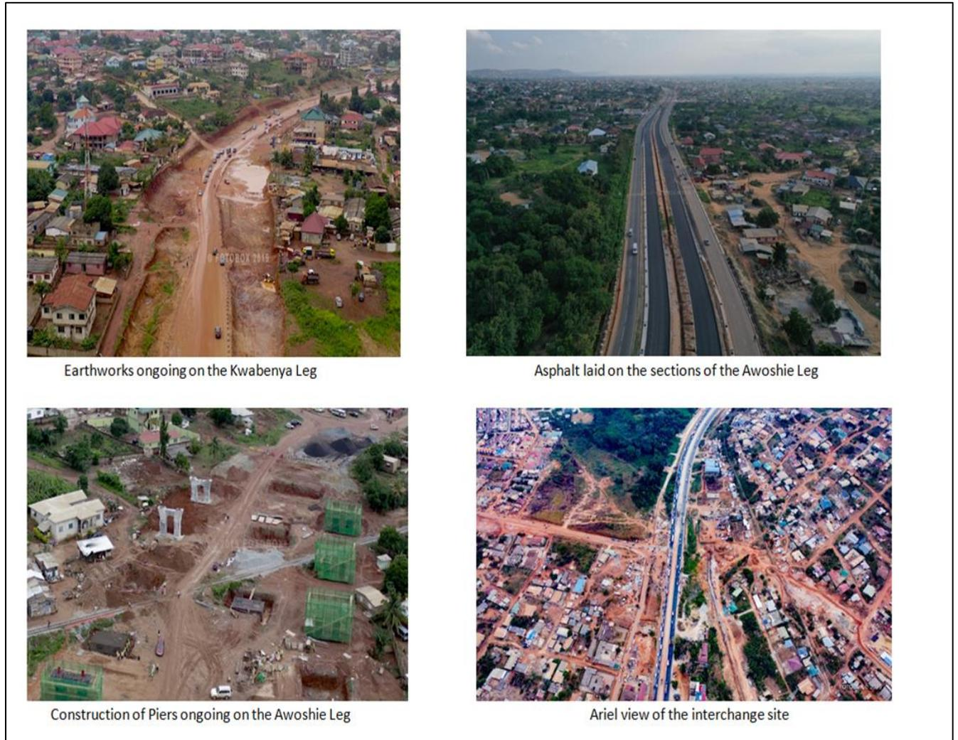
**Figure 1: Status of ongoing works at the Pokuase Interchange as part of the Accra Urban Transport Project**
