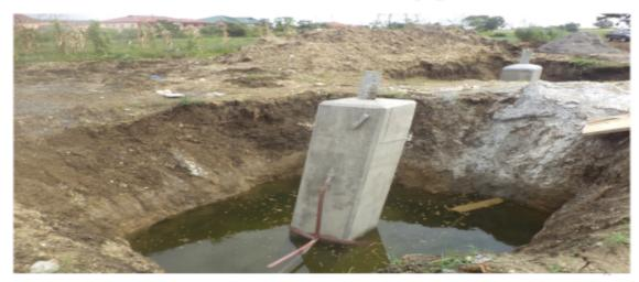
Casting Of Reinforced Cement Concrete Pad For Tower BT4/6 Foundations And Chimney For Tower BT4/1:-Volta-Achimota-Mallam Upgrade
