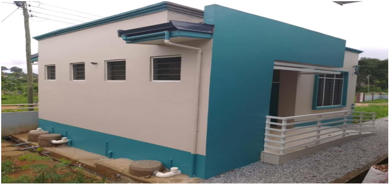
COMPLETION OF 3No. REPRODUCTIVE HEALTH CLINIC AT KOJOKROM, DIABENE, ESSIPONG.
