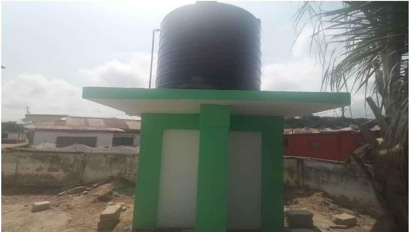
CONSTRUCTION OF 40No. BOREHOLE FOR SELECTED COMMUNITIES IN THE METROPOLIS
