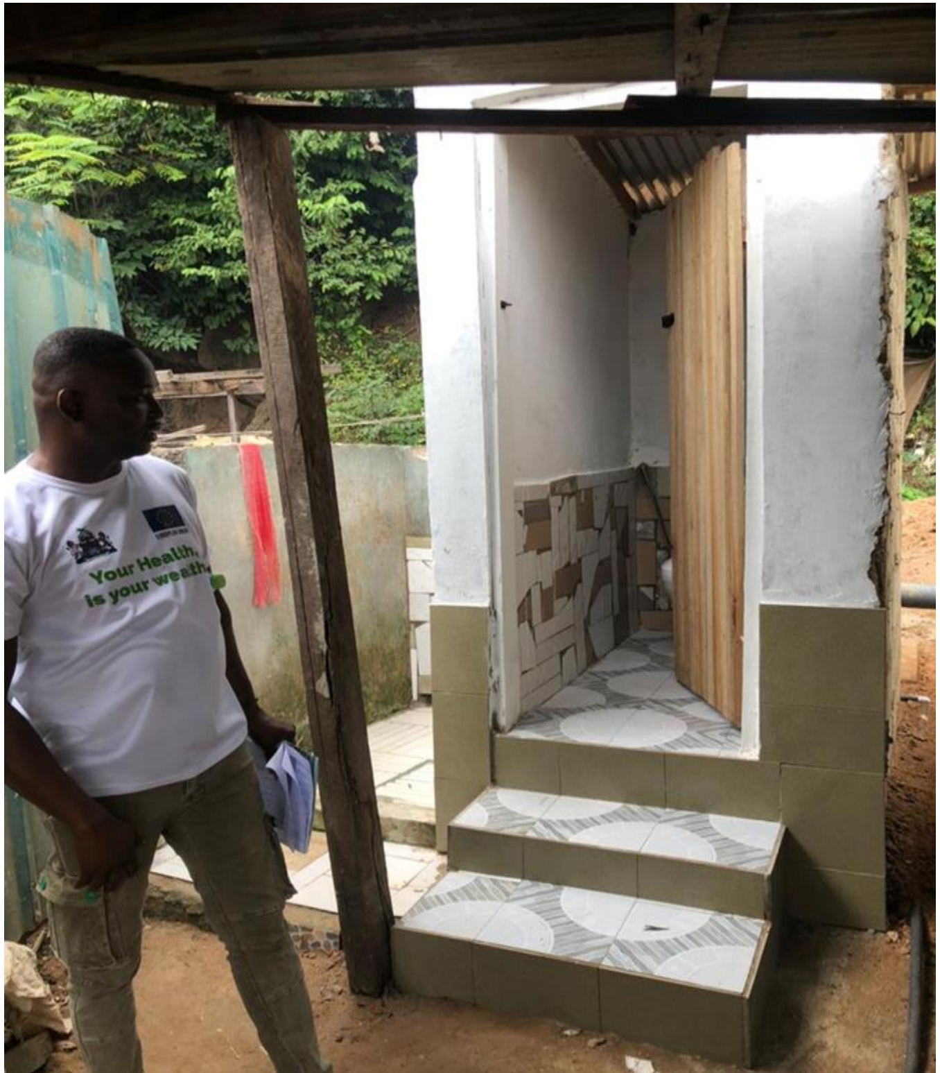
COMPLETED THE FINAL 200 th . BIOFILL DIGESTER TOILET FACILITY (400 UNITS IN ALL)
