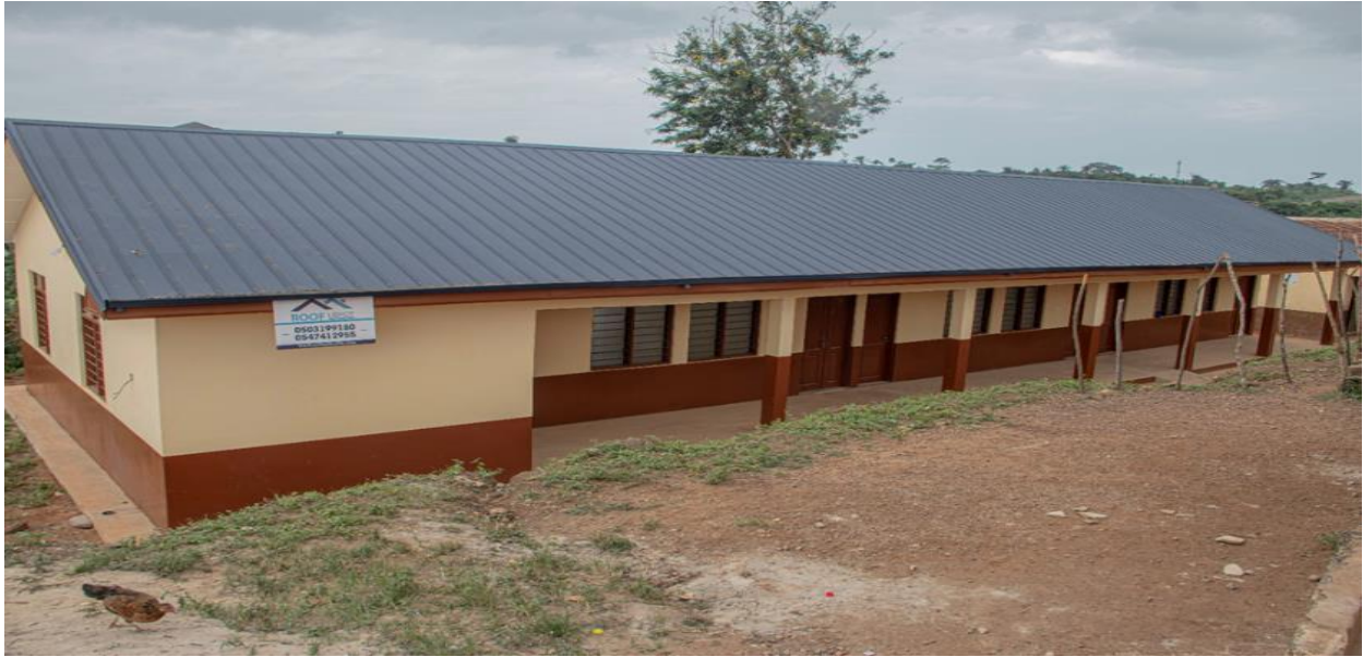
CONSTRUCTION OF 1 NO. 3 UNIT CLASSROOM BLOCK WITH ANCILLARY AT INCHABAN NKWANTA.
