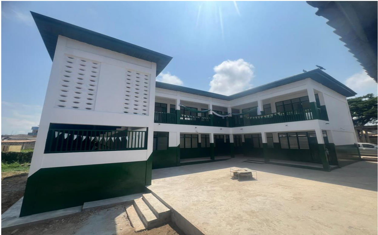
CONSTRUCTION OF 3 UNIT CLASSROOM BLOCK WITH OFFICES AND STORES AT BISHOP ESSUAH -TAKORADI.
