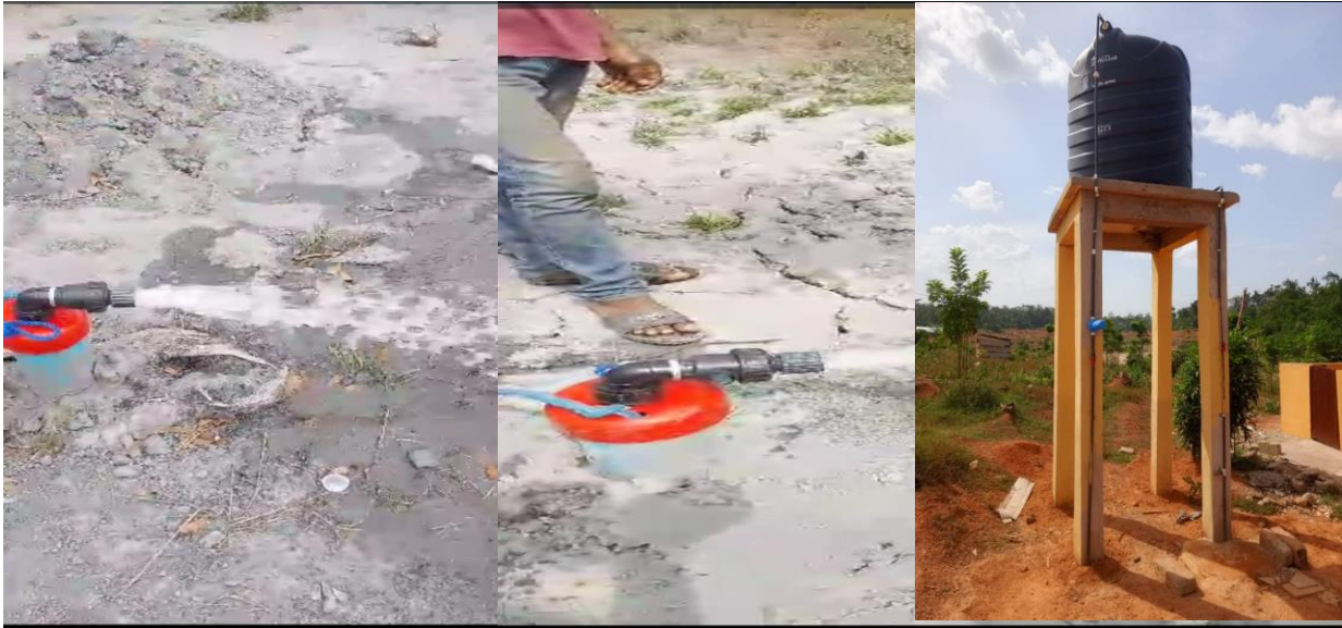
Completed the Construction of 2 NO. Borehole at Manso Amenfi Technical Institute
