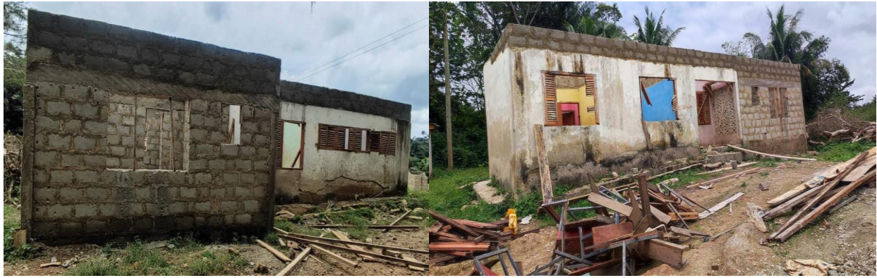
Renovated of Teachers Quarters at Dwirigum
