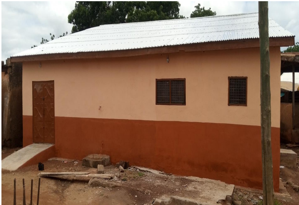
Figure 2: Renovated and Furnished 1No. Meat Shop at Yabapeling-Fumbisi
