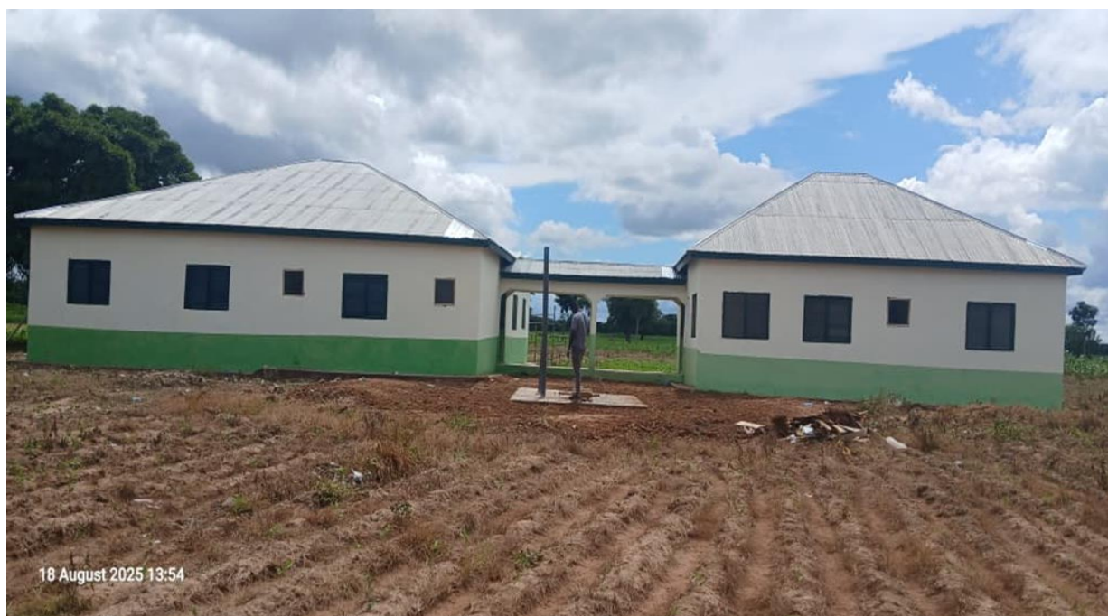
Figure 3: Completed and furnished 1No. CHPs compound at Tuedema
