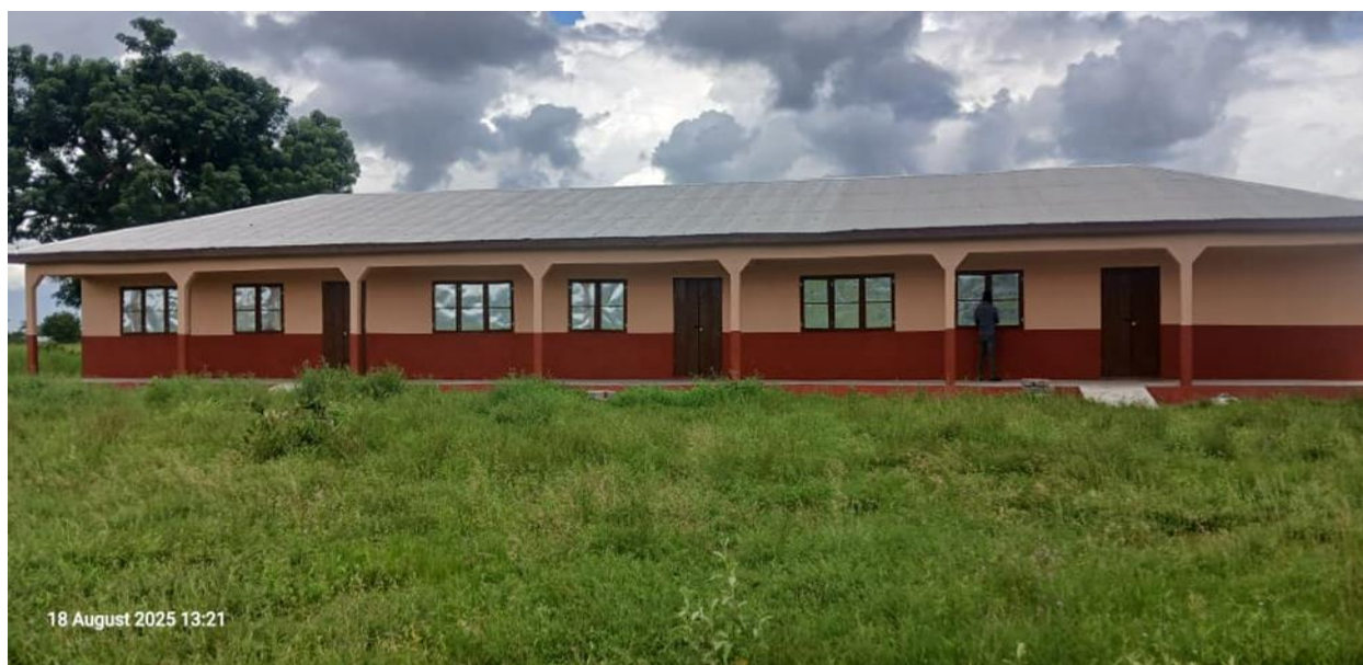
Figure 4: Constructed and furnished 1No. 3-Unit Classroom block with ancillary facilities at Batuisa
