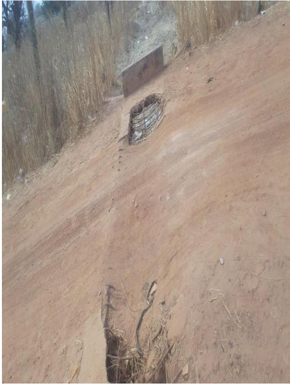
Constructed 3No. 1.2M double pipe culverts and 2No. 3x2M box culverts with earth fillings at Catholic Church Road-Soe
