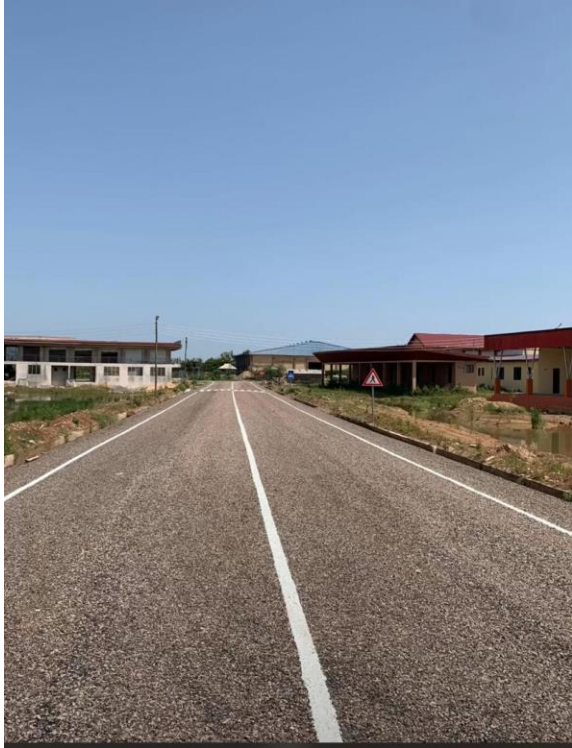
Constructed 2.52km Length of Road Network, 5.4km Length U-drains, and 2no. 1.2m and 9no. 0.9m Culverts at the Mechanics Enclave
