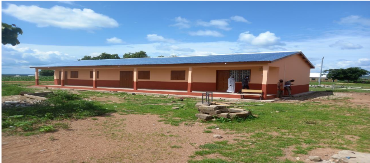
Constructed 1No. 2 Unit Classroom Block with office and store at Yalugu
