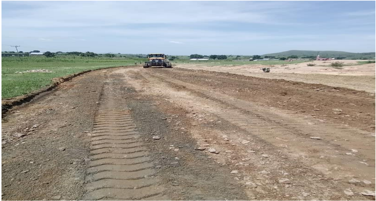
Constructed access feeder road from zuawesi to Bansi
