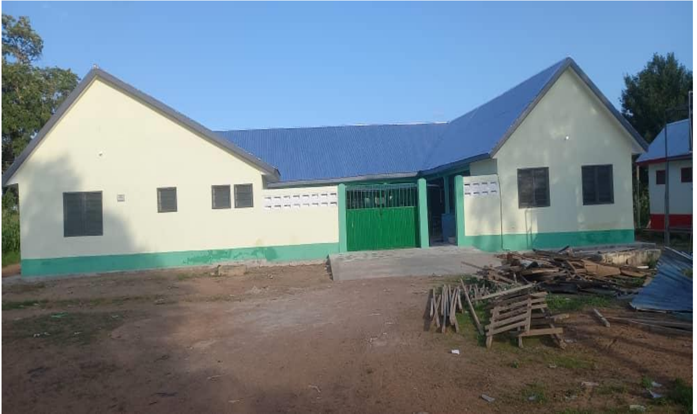
Constructed 1NO. CHIPS AT BANSI
