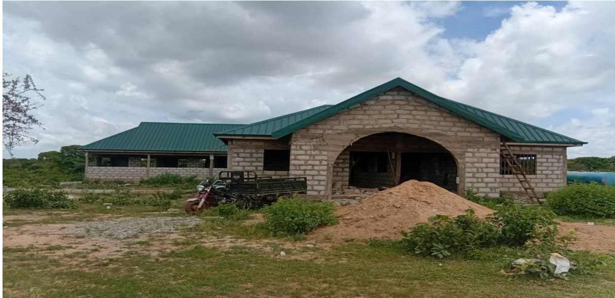
Constructed health administration block at Avoundago
