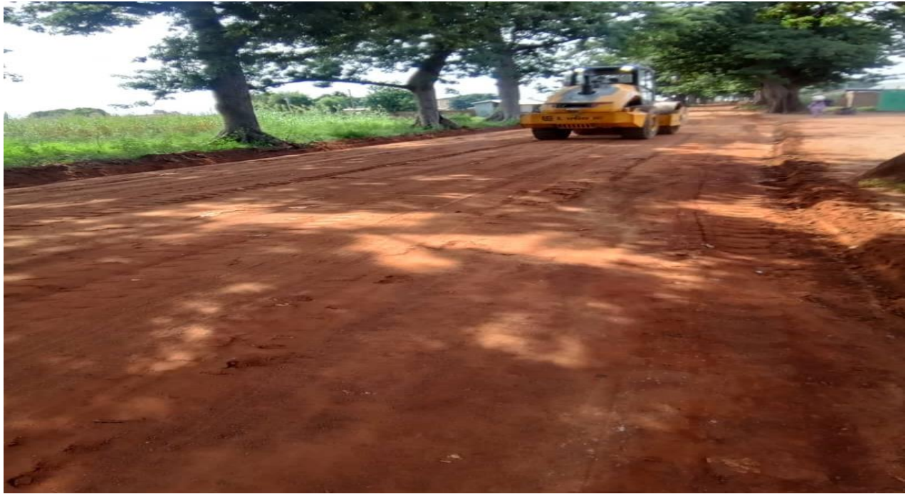
Reshaped feeder road from zawse to GES Junction
