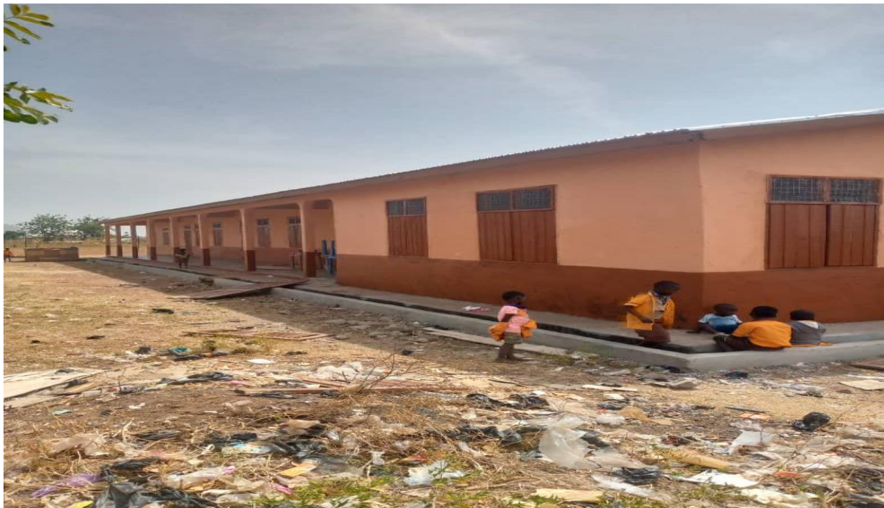
Constructed 1No. 6-unit classroom block at Bansi with furniture
