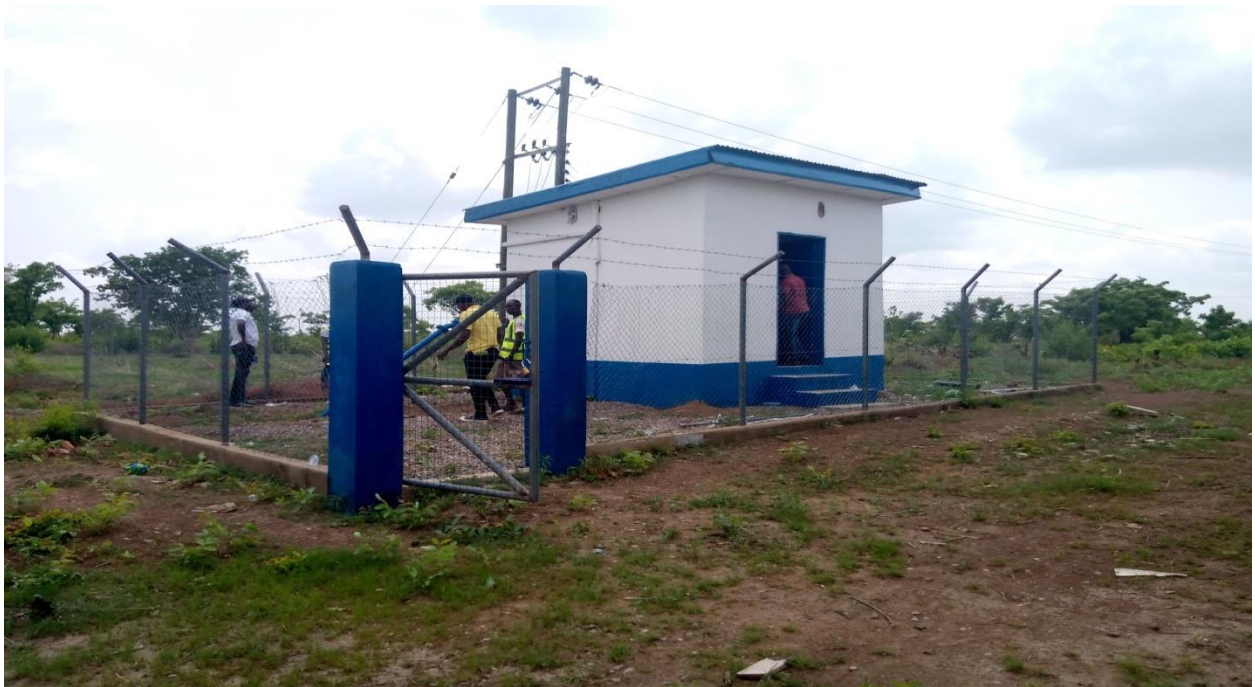
Kpalbe Water system
