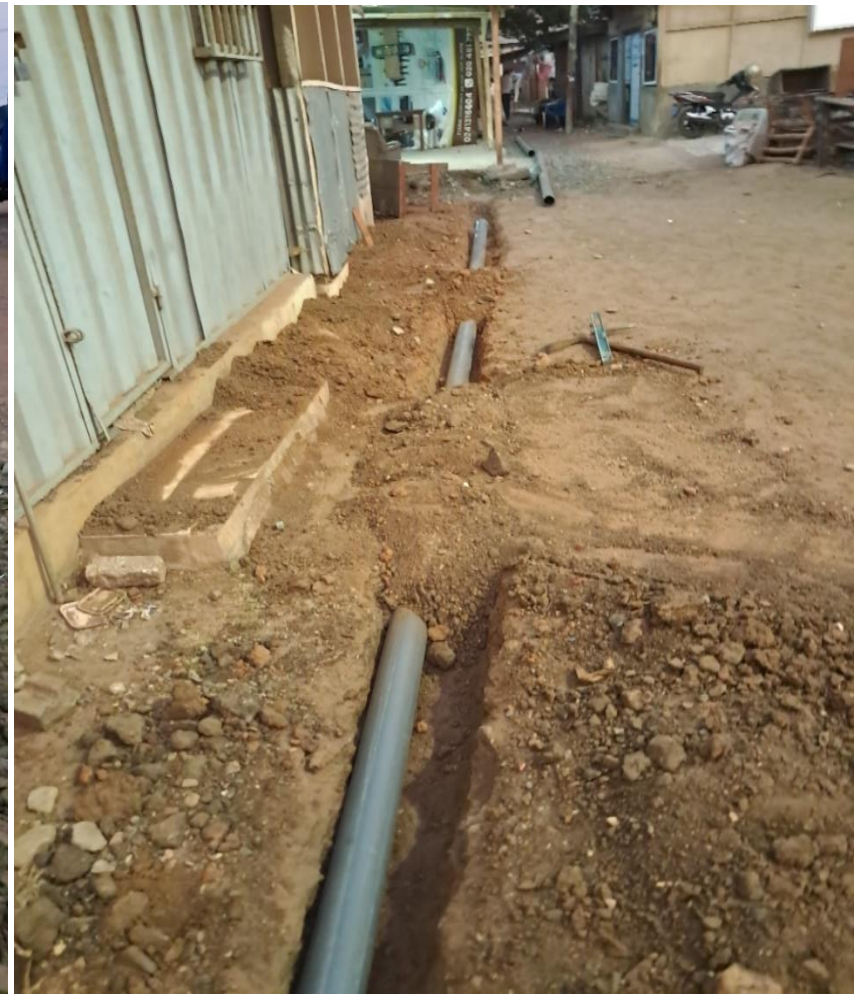
Replacement of broken sewer pipes and Construction of intermediary manholes at Community 5 Market and Community 5 B road Area
