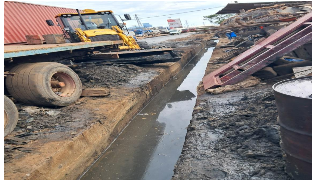
Desilting and dredging of drains from Yara Ghana to behind the Mexico School and inner drains at Community 2
