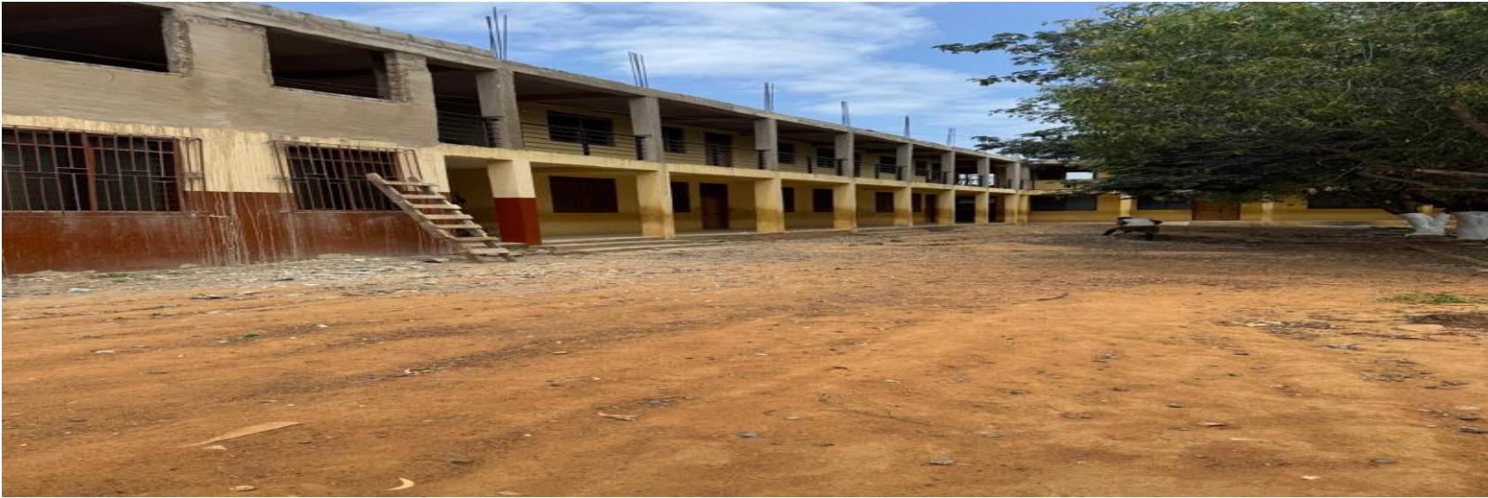
CONSTRUCTED 12-UNIT CLASSROOM BLOCK AT STAR BASIC SCHOOL (PHASE II)
