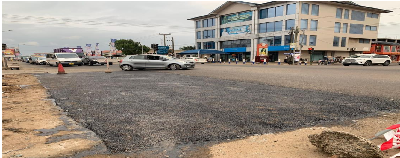
EMERGENCY CONSTRUCTION OF ACCESS SLAB AT ECOBANK JUNCTION-TEMA WEST MUNICIPALITY.
