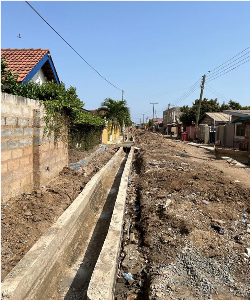
CONSTRUCTION OF U-DRAINS WITHIN THE MUNICIPALITY
