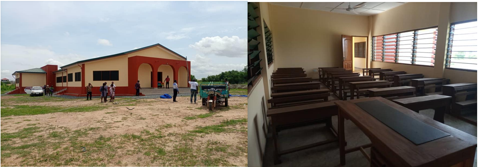
CONSTRUCTED 6 UNIT MODERN CLASSROOM BLOCK AT ADJEI KOJO
