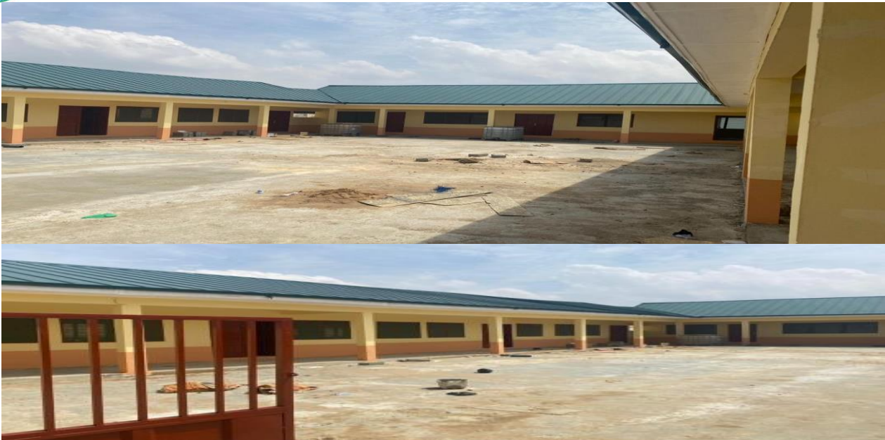
CONSTRUCTED 1 NO. 6-UNIT CLASSROOM BLOCK AT PADMORE SCHOOL
