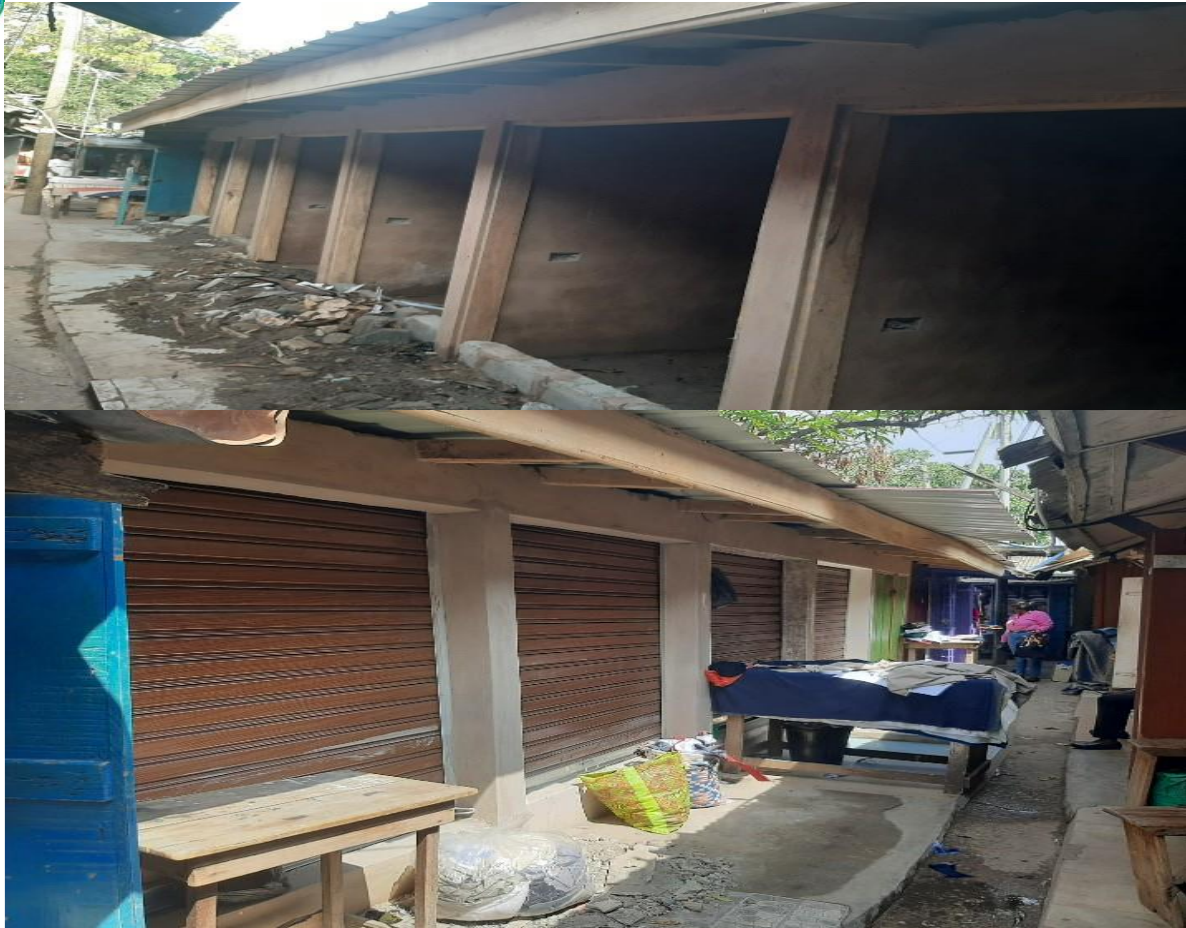
RECONSTRUCTED 7NO. STALLS AT COMMUNITY ONE MARKET
