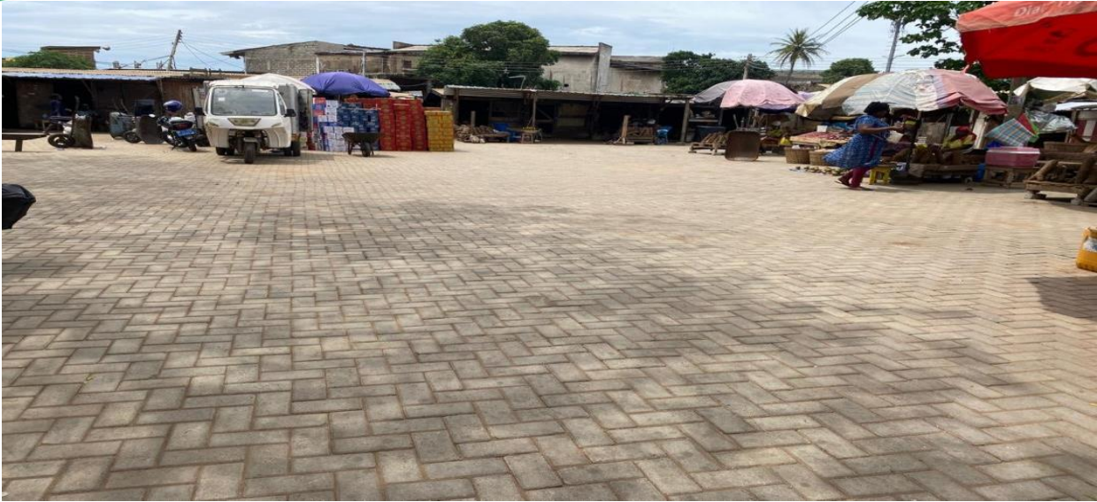
REDEVELOPED (PAVING WORKS) YAM MARKET AT TEMA COMMUNITY 1
