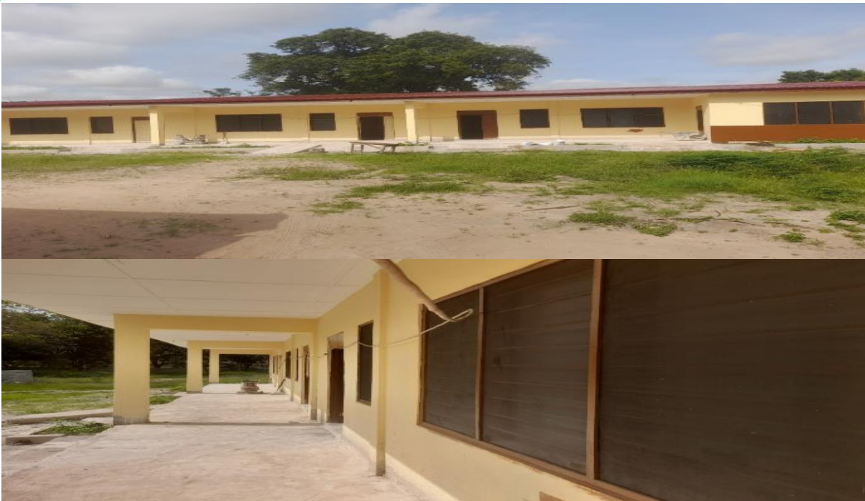
CONSTRUCTED 1 NO. 3-UNIT CLASSROOM BLOCK AT COMMUNITY 8 NO. 2
