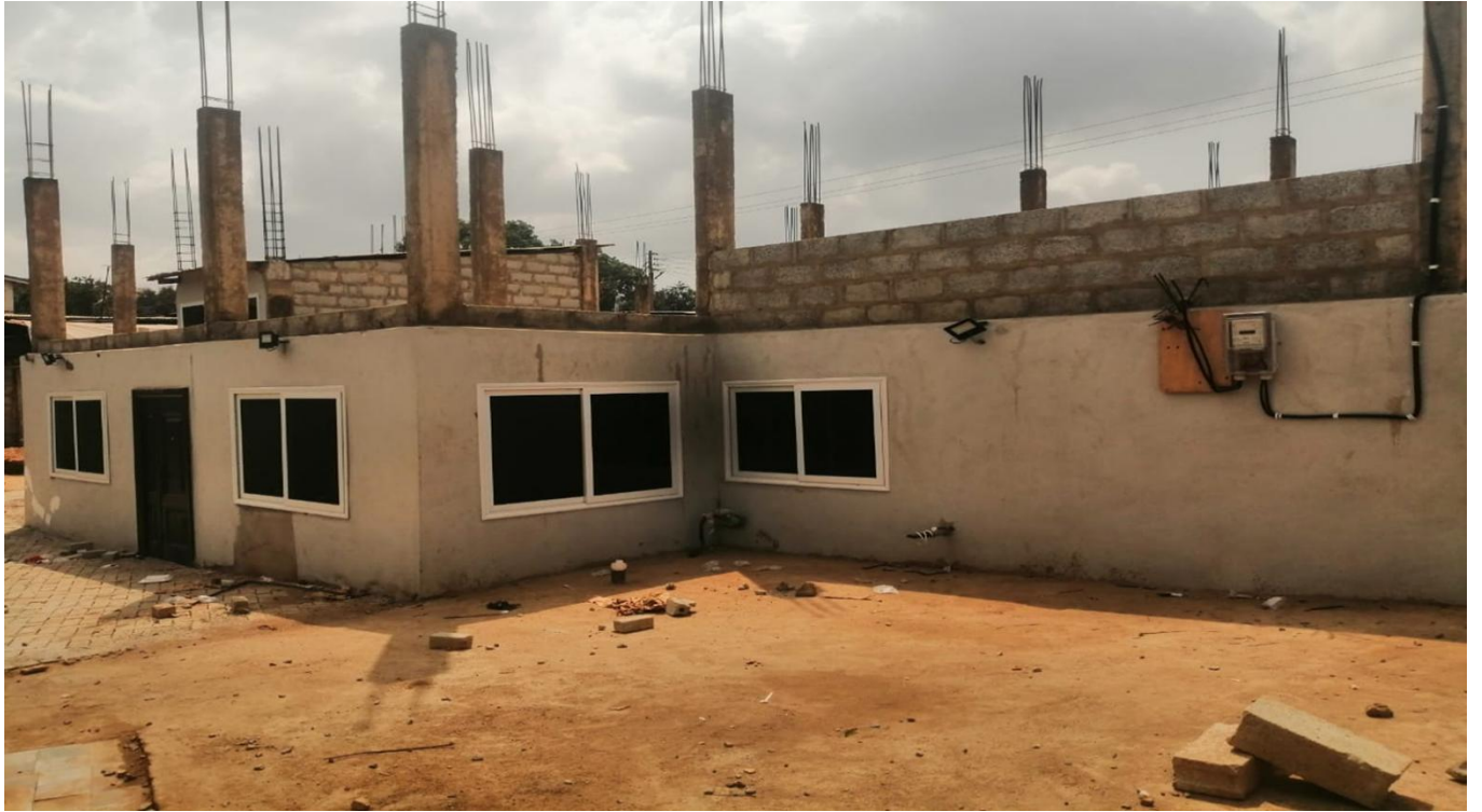
Completed Basement of Clinic at Christian Village
