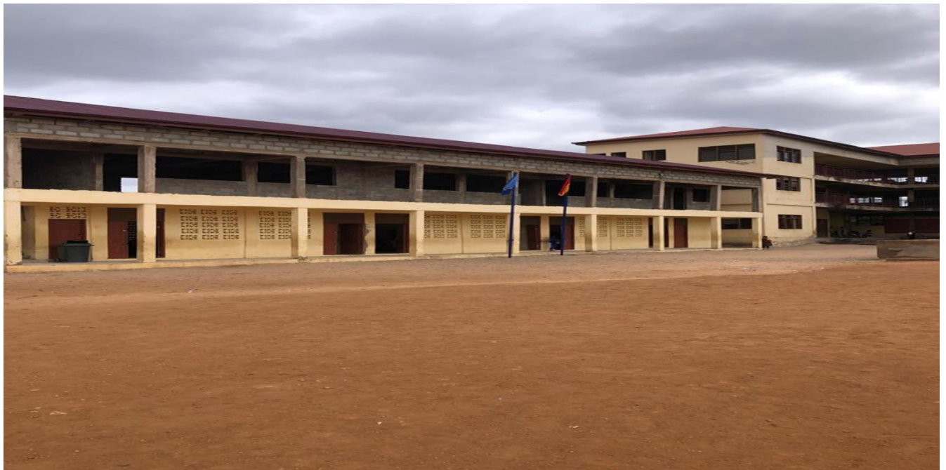
First Floor Of 2 Storey 3-Unit Class Room Block And I.C.T Library
