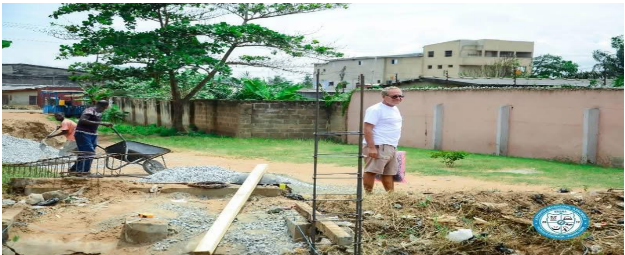
Dredging works across the municipality
