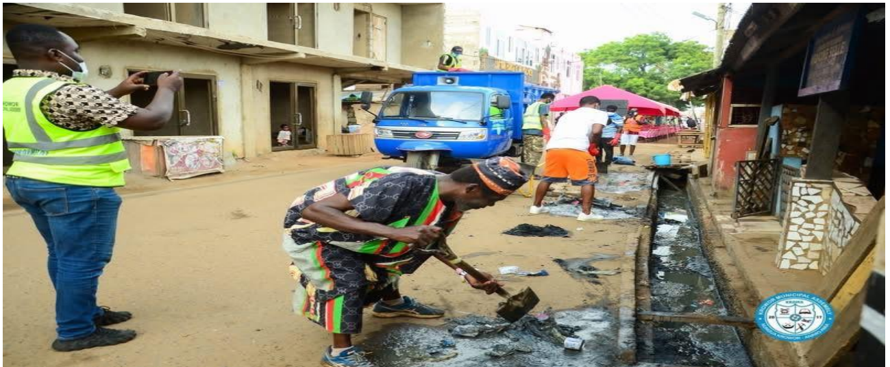
Desilting of drains in the Municipality
