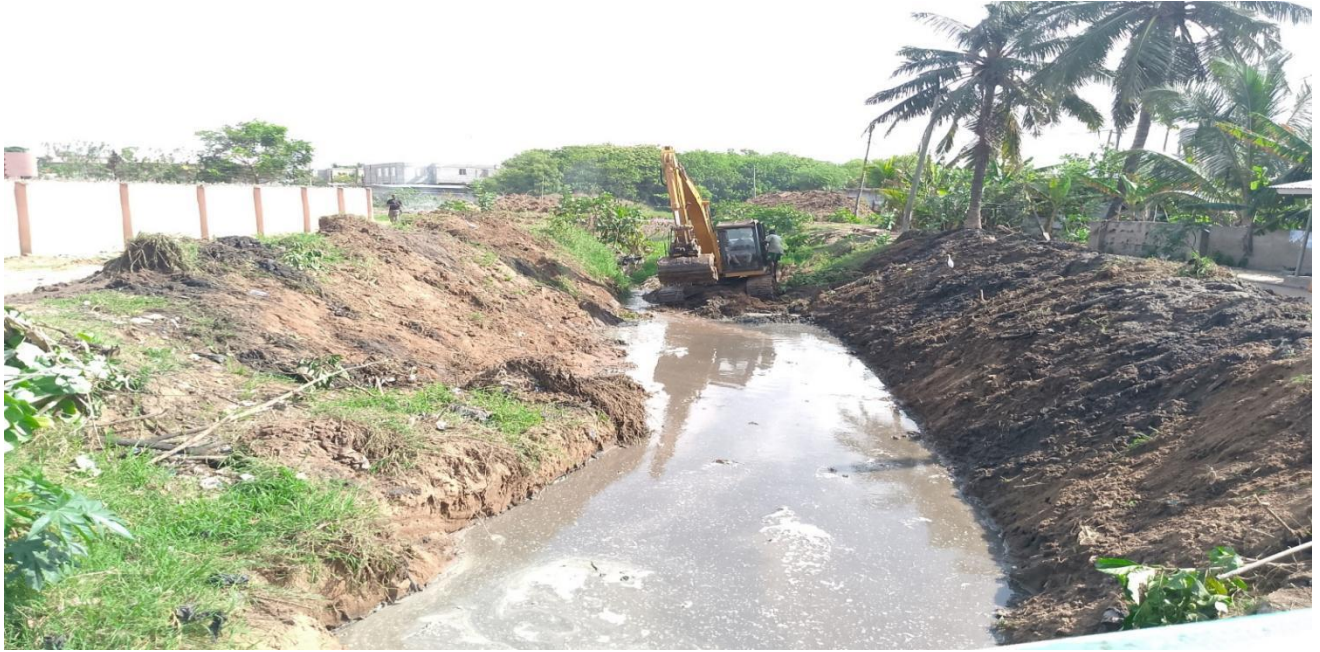
Dredging of Awikonaa from AG Church to Old Kasapreko (During)
