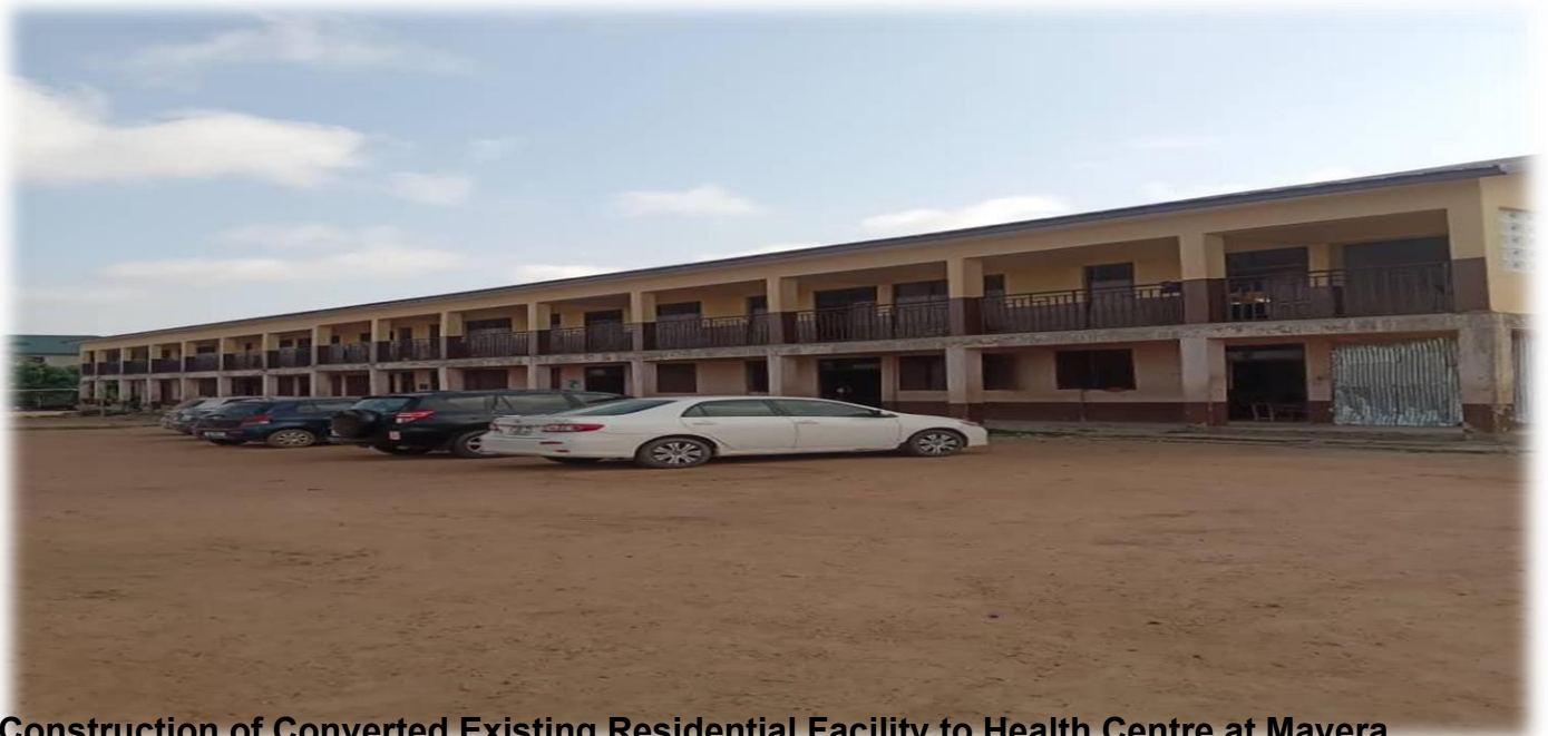
Construction of Converted Existing Residential Facility to Health Centre at Mayera
