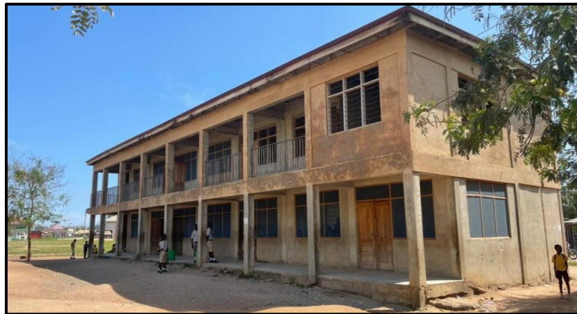
Completion of 1 No. 3 unit classroom block at Avornyokope Classroom Block at Ashalaja
