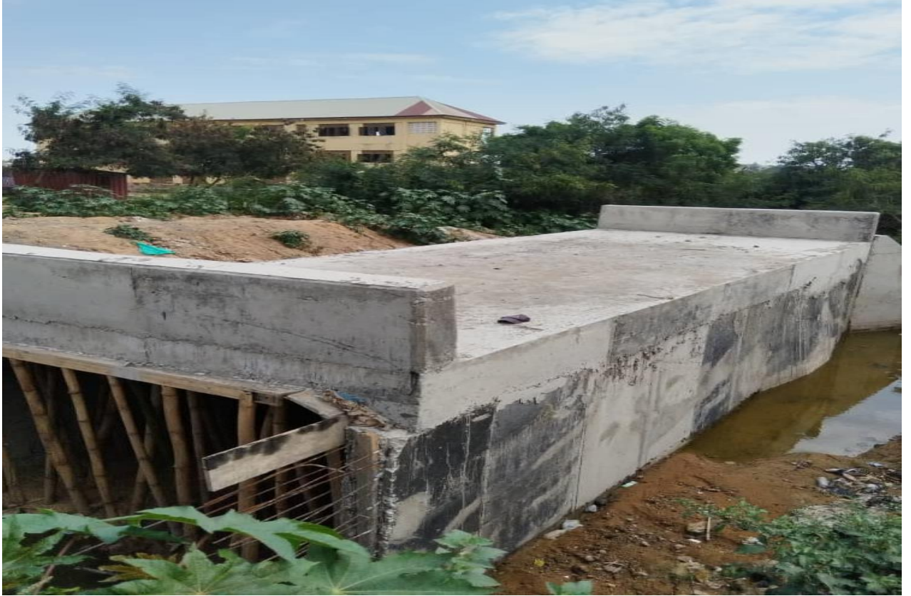
Picture 5: CONSTRUCTED U-DRAIN AT ANYAA DEEPER LIFE LINK
