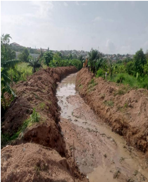
Picture 7: DREDGING WORKS AT LAFA STREAM, KWASHIEBU
