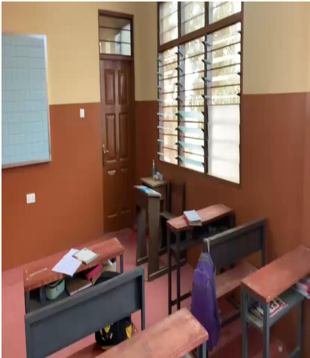
Picture 2: CONSTRUCTION OF 6-UNIT CLASSROOM BLOCK AT GREATER D BASIC SCHOOL (PHASE I)
