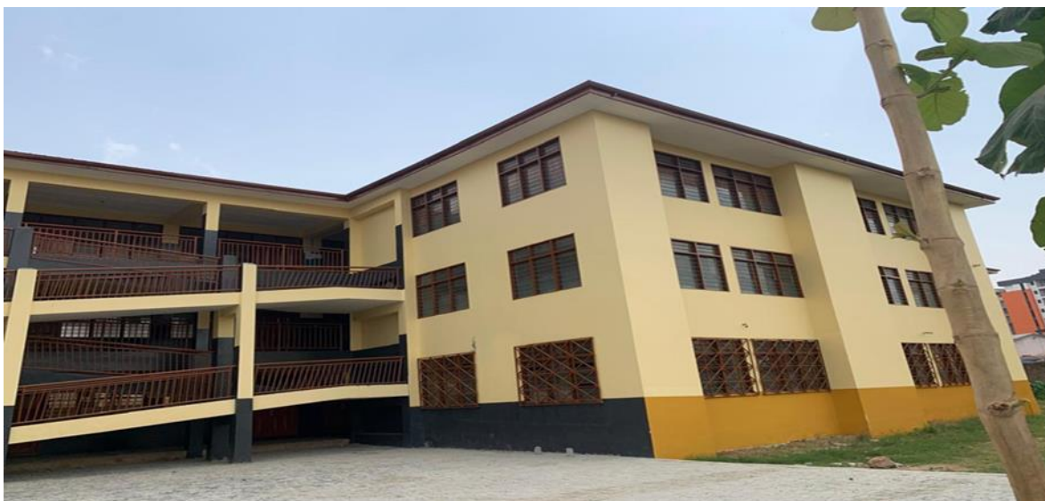
Picture 3: Renovated Roman Ridge M/A Basic school (IGF)
