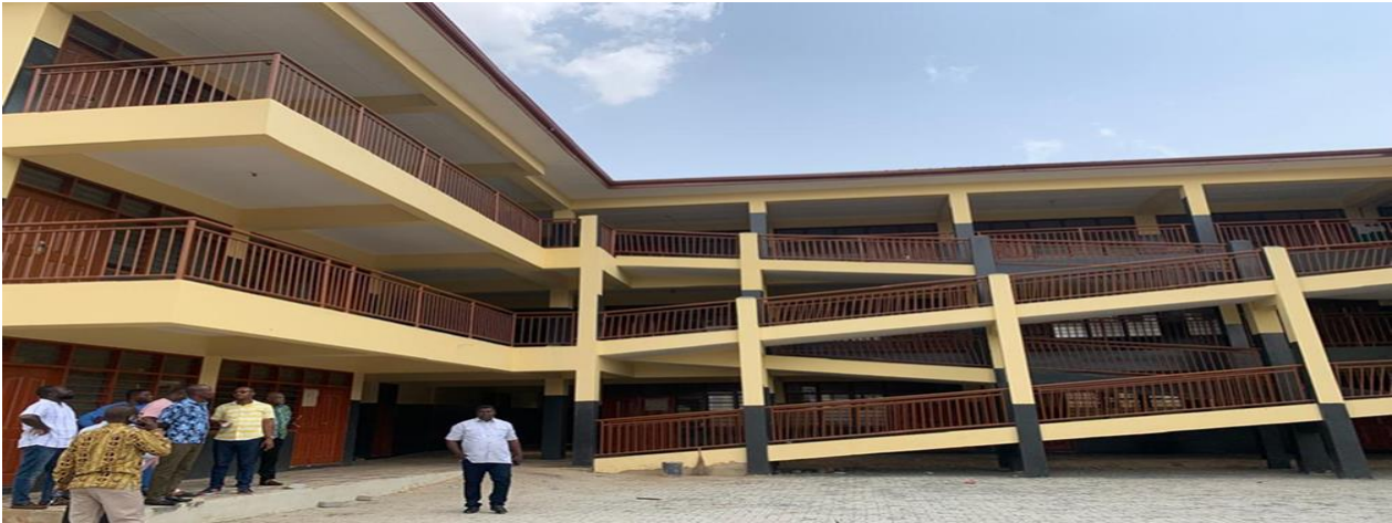
Picture 4: Renovated Roman Ridge M/A Basic school (IGF)
