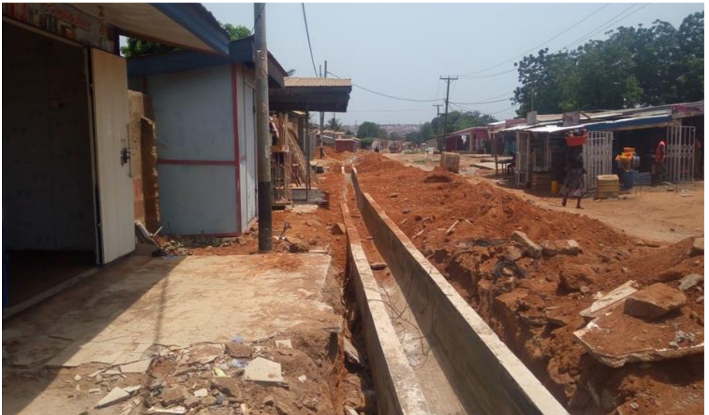
REHABILITATED ADJIRINGANOR SIXTY-NINE (69) AREA ROADS (3.09KM)
