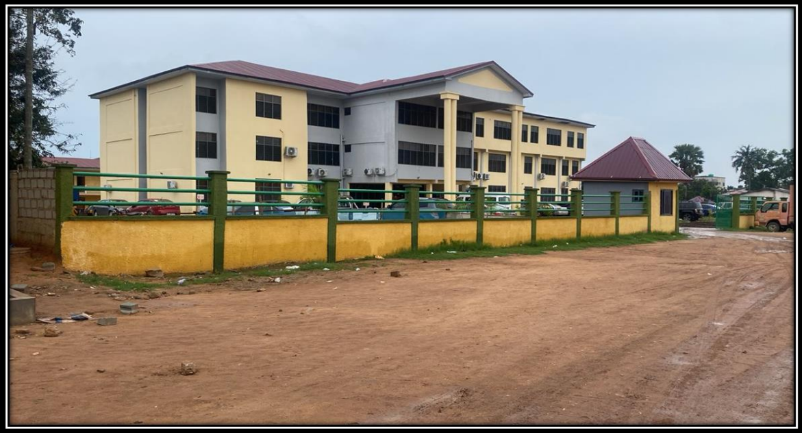
Constructed external walls and gatehouse at the Municipal office complex
