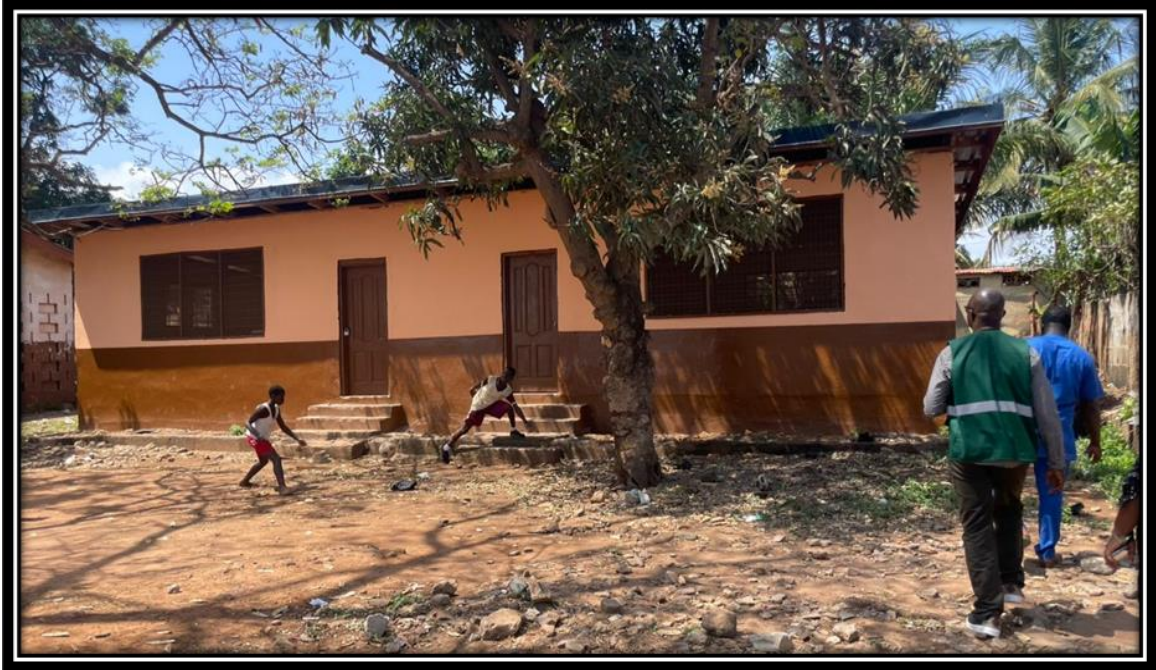
Renovated Classroom Block at L/B 1 School
