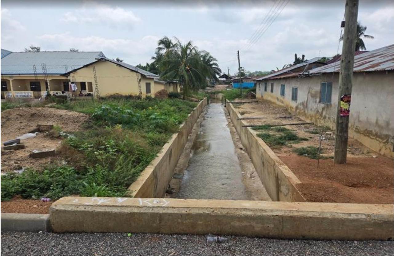
Constructed 1.1km rectangular concrete storm drain (2.5*2.5m) at James Town, Asamankese
