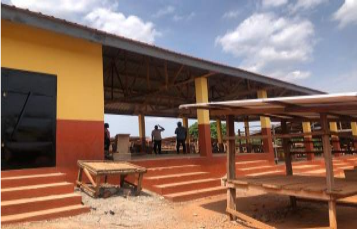
Constructed 1 No. 20 Unit Market Shed with 2No. Warehouse at Sekesua
