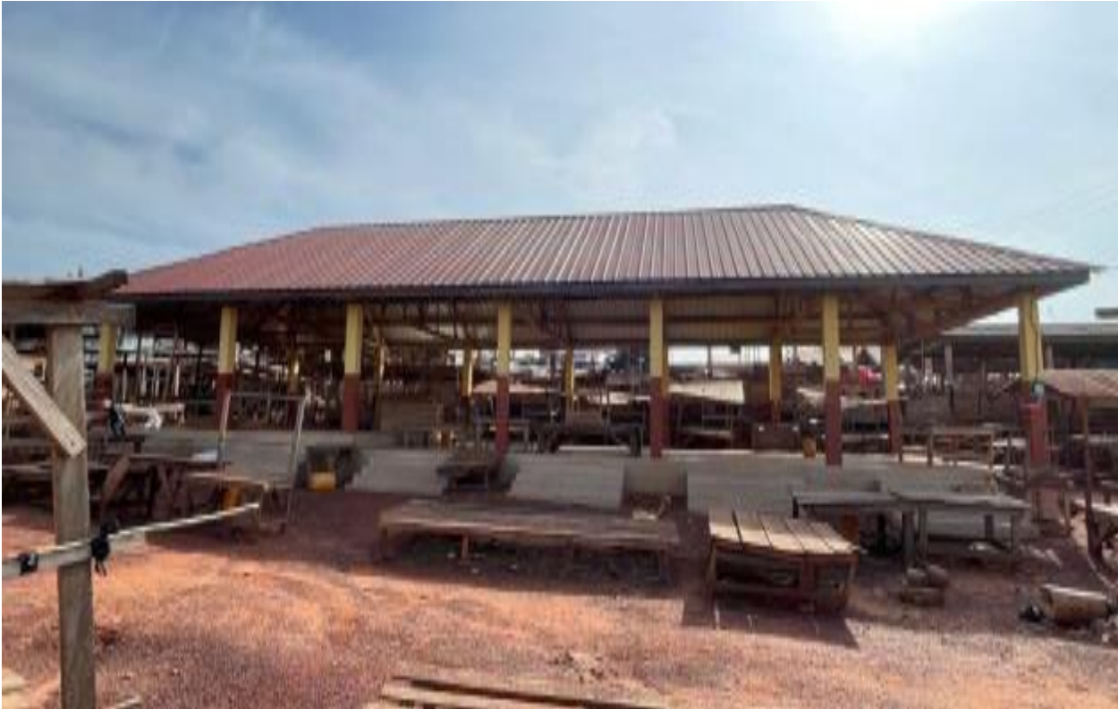
Constructed 1 No. 24 Unit Market Shed At Asesewa
