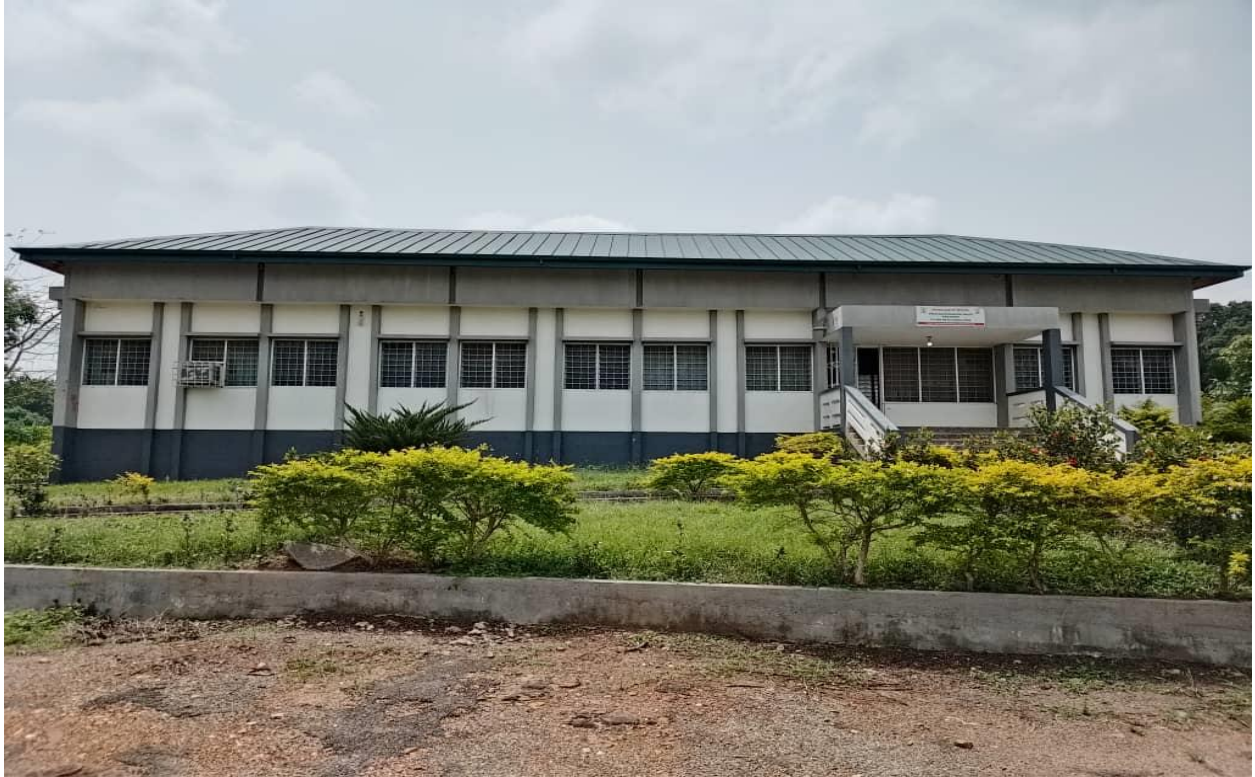
CONSTRUCTED A POLICE STATION AT ADAWSO
