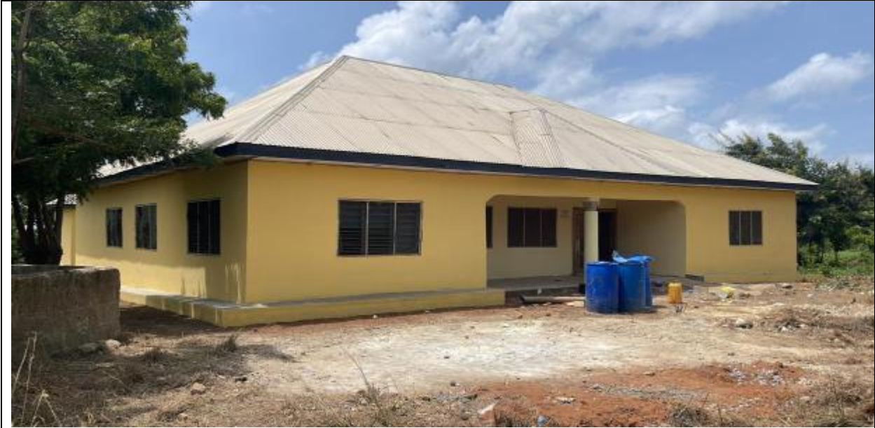
Rehabilitation of Bokuruwa CHPS compound & Nurses Quarters (75% Completion)
