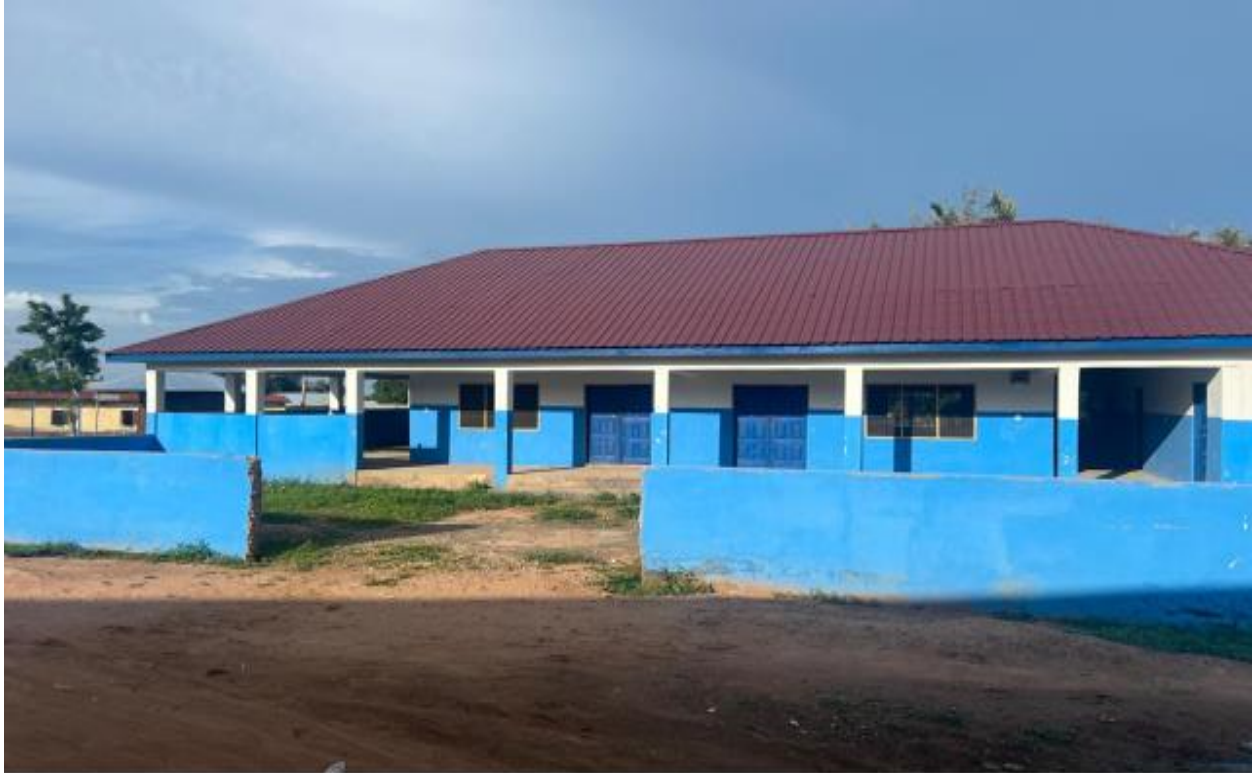
Fig 16: Constructed 2-Unit Classroom Block at Donkorkrom (90% Complete)
