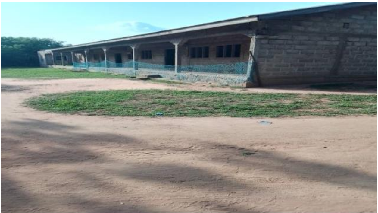
Fig 17: Constructed 3-Unit Classroom Block at Sihu Norfegali (75% Complete)
