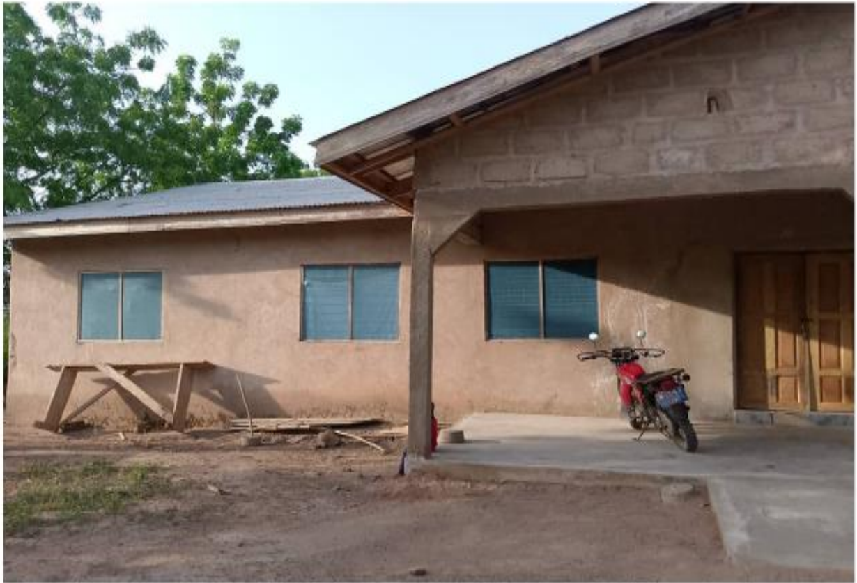
Fig 15: Constructed 1No. CHPS Compound at Kokrobuta (90% Complete)
