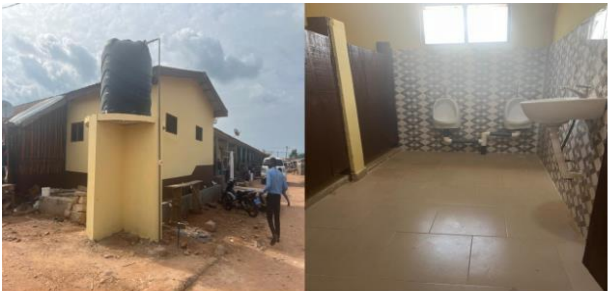
Fig 19: Constructed 6No.Toilet And Urinal at Donkorkrom Market
