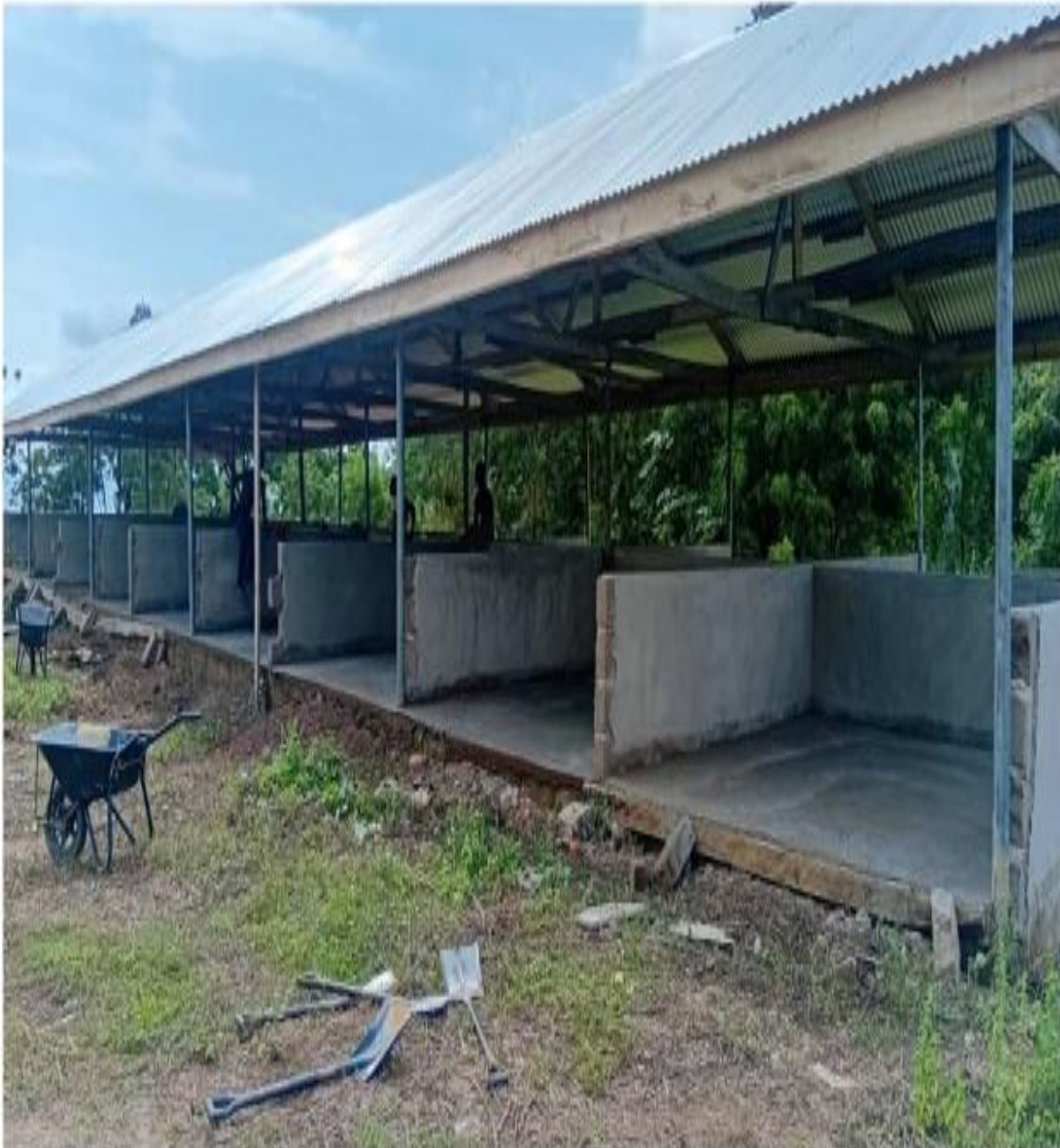
Fig 20: Constructed 20No. Satellite Market Stalls At Agordeke (90% Complete)
