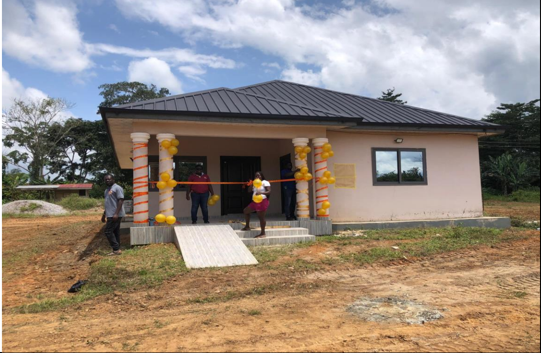
Constructed Training centre with ancillary facilities for Akyem Awenare
