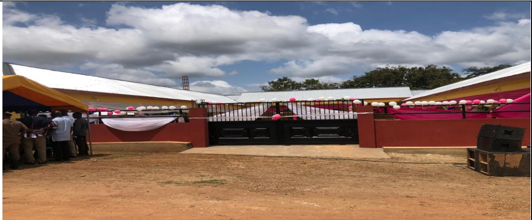
Completed 1 no. Community Durbar ground at Erkoso Akwadum
