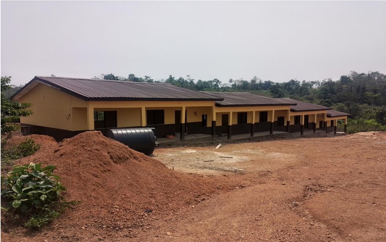
Constructed 1no. 3-Unit Classroom block at Apamso
