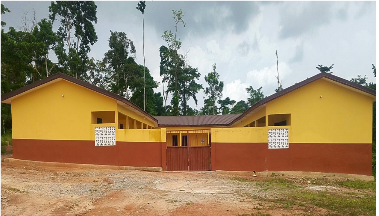
Constructed 1no. 6-Unit Classroom Block at Ahumtem
