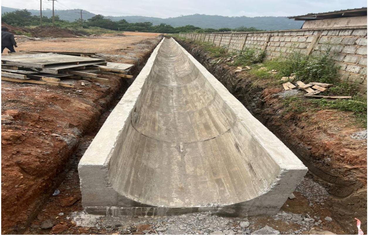
Construction Of U Drain at Kronum Market
