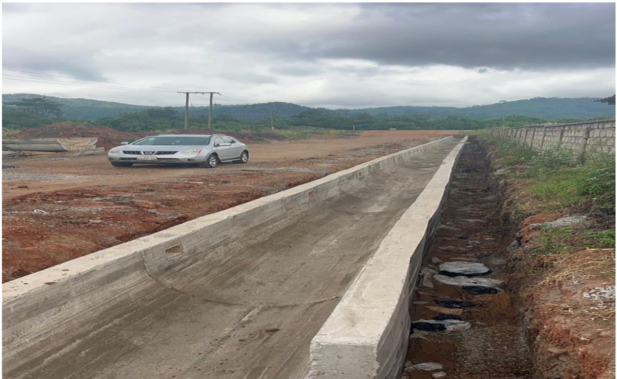
Construction Of Storm Drain at Abusuakuruwa
