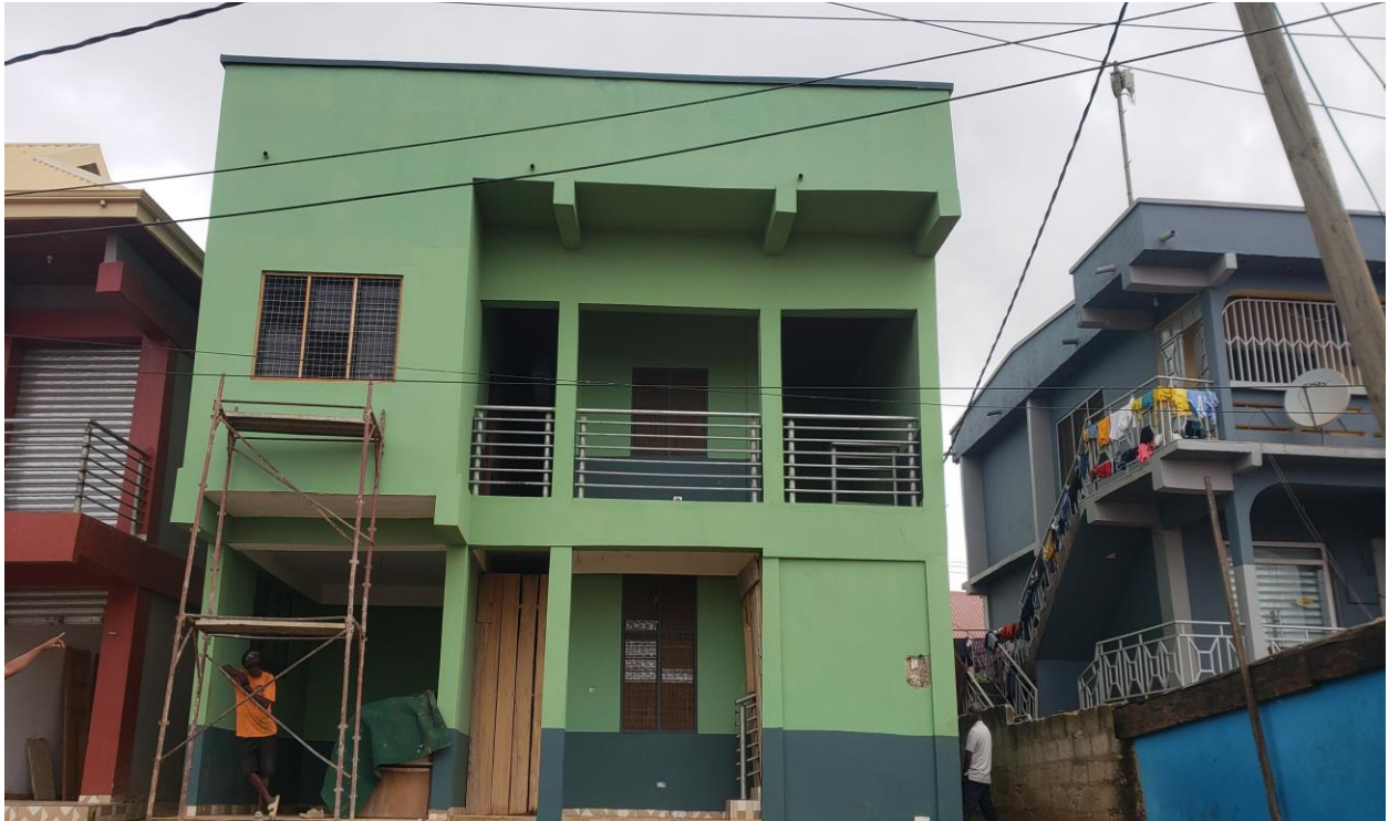
Completed construction of Ambulance Bay at Tarkwa-Maakro
