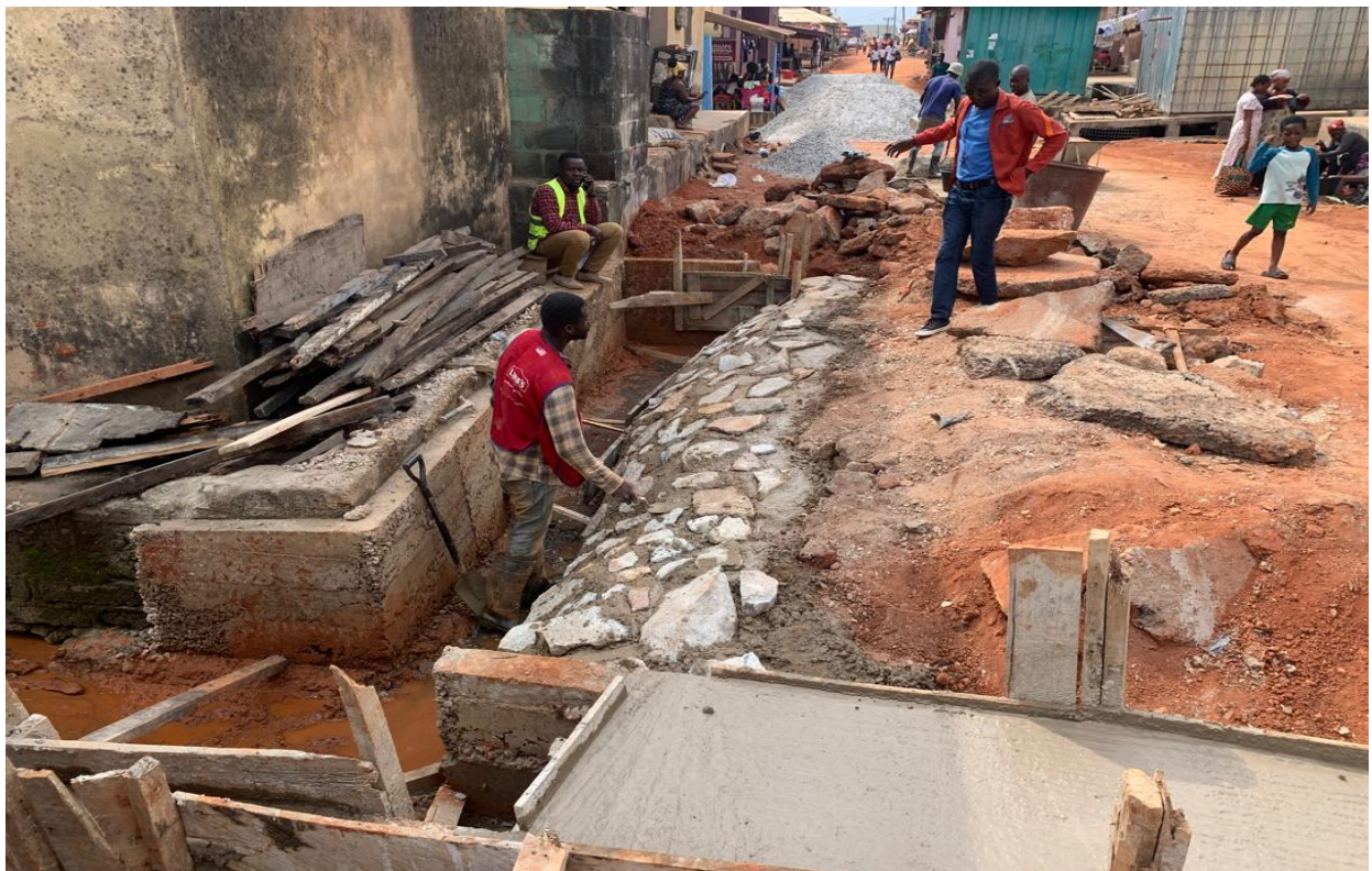
Construction Of U Drain at Kronum Market
