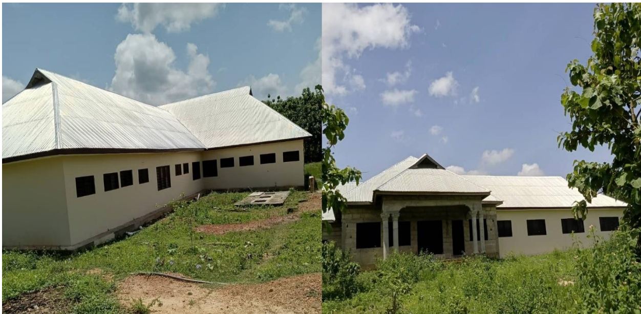
Completed Health Center at Nkwankwanua (Phase 1)
