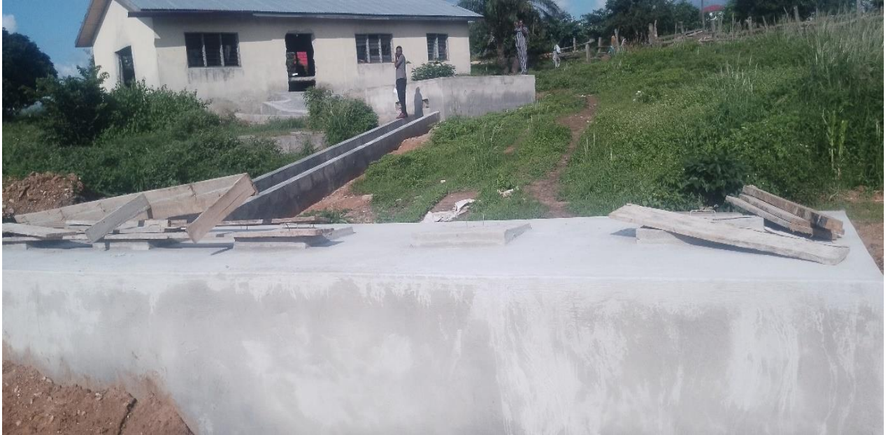
Figure 10: Rehabilitation of Slaughter House Nsuta -IGF
