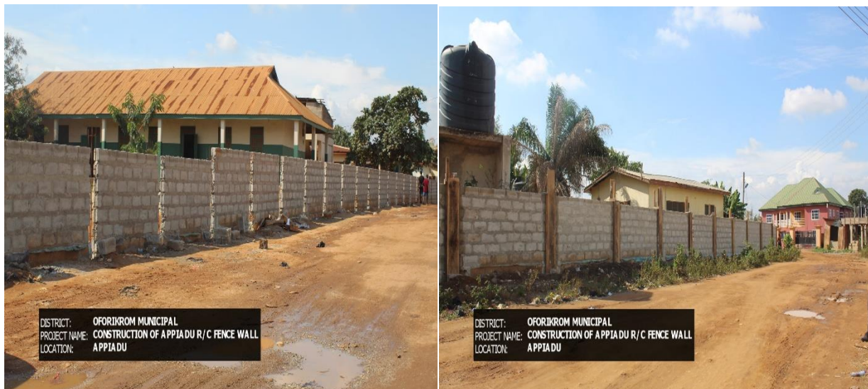
Constructed 674M Fence Wall at Appiadu R/C School
