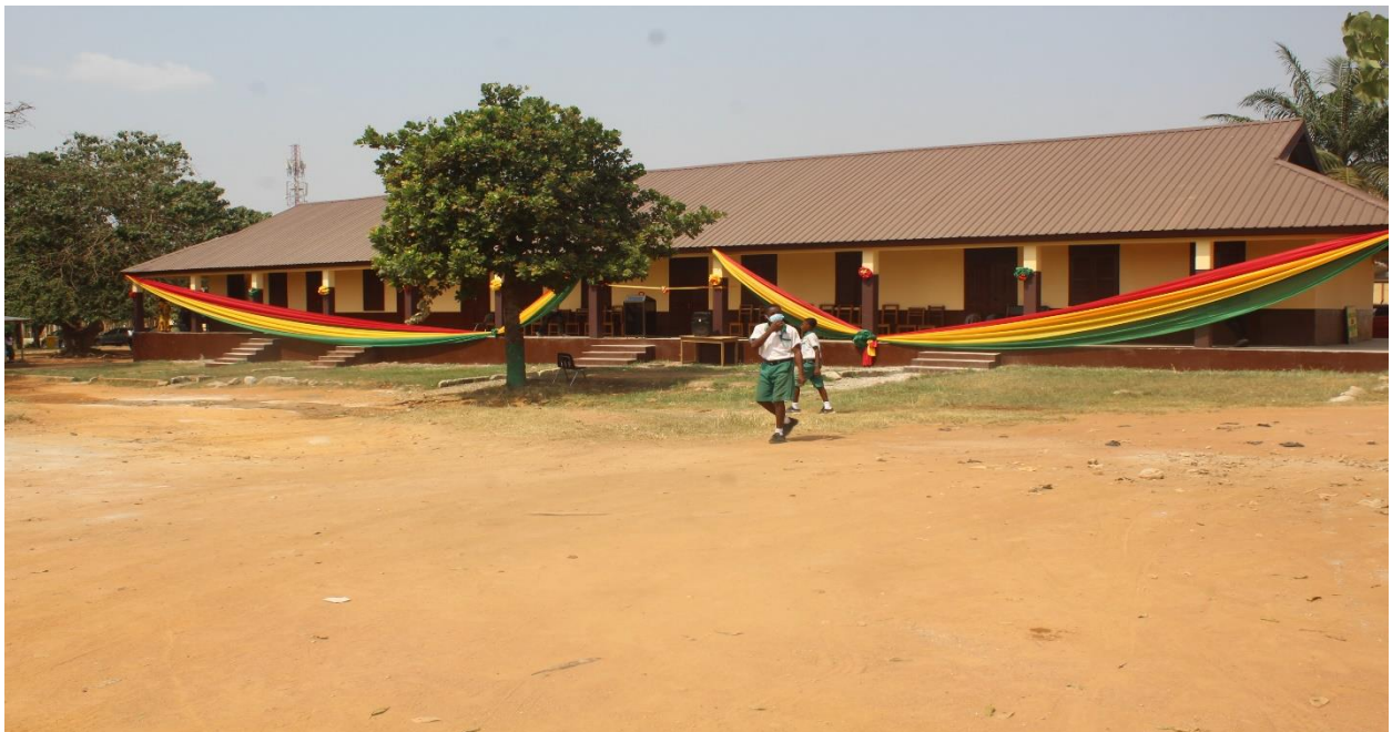
Renovated 1No. 3-Unit Classroom Block with Office and Store at Kotei R/C School
