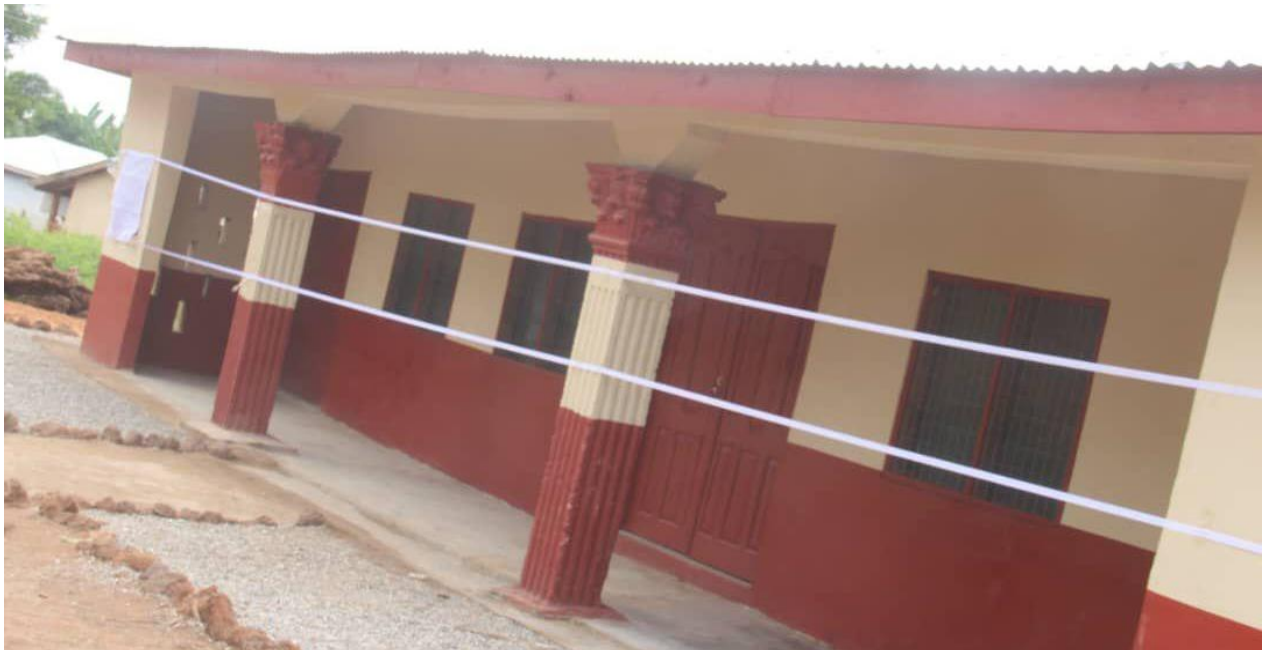
1 No. 2 Unit Classroom Block constructed at Nnobem
