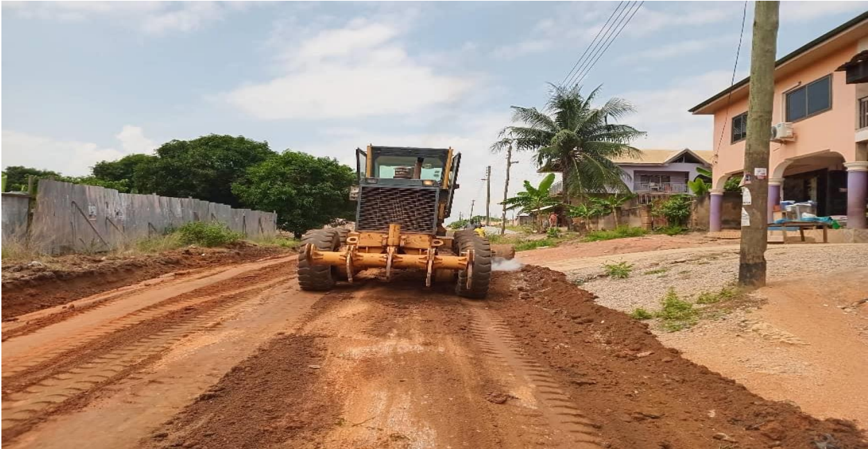
RESHAPED ROAD AT APATRAPA 6KM(DRIP-DACF/IGF)
