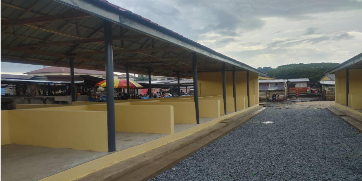
CONSTRUCTED 4NO.10 MARKET STALLS AT ASUOYEBOA PHASE I(DACF-RFG)
