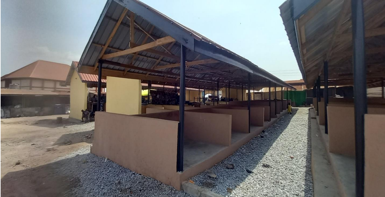
CONSTRUCTED 4NO.10 MARKET STALLS AT ASUOYEBOA PHASE II(DACF-RFG)
