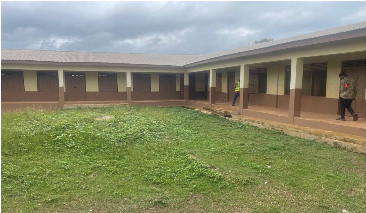
Completed 1No. 3-Unit Classroom block at Saakrom
