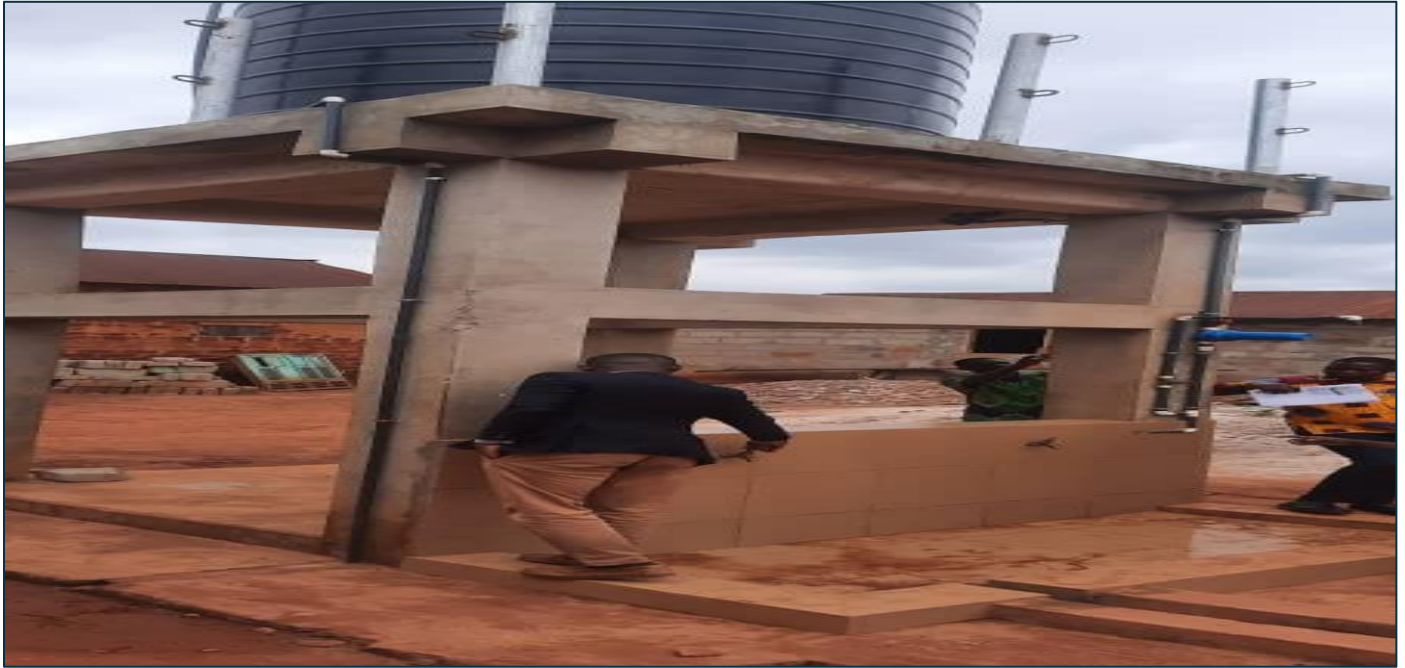
Completed 1no. Mechanized borehole at Nsuta
