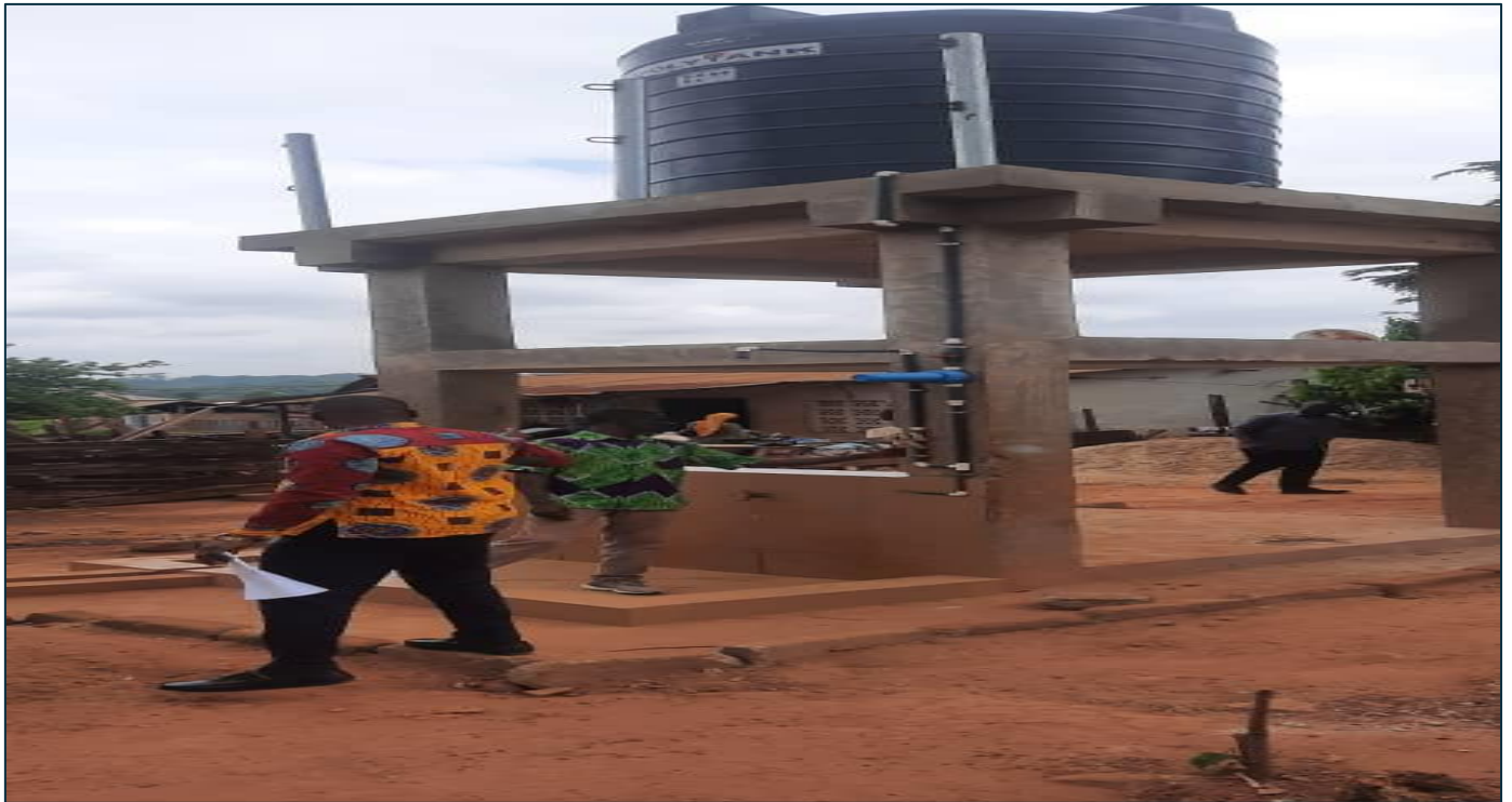
Completed 1no. Mechanized borehole at Abesewa
