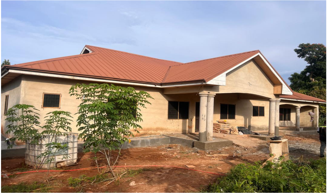
Completion of 1No. CHP Compound at Mehame
