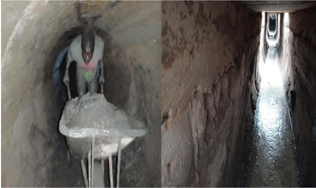
Desilted of 500m Pipe Culvert and U – Drain at Ofankor Roundabout
