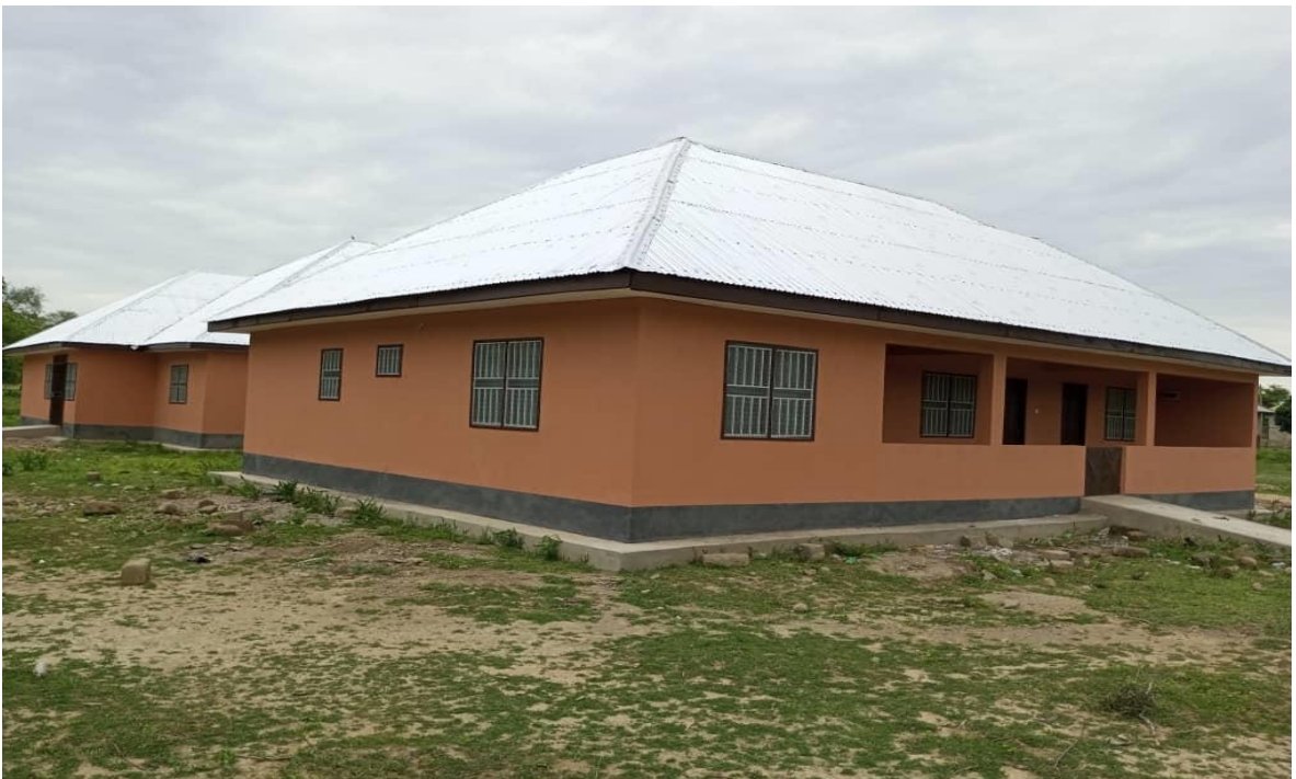
Constructed 1No CHPS Compound at Kumbosigo
