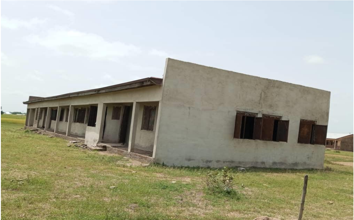
Construction of 1No 3-Unit classroom block at Dubila
