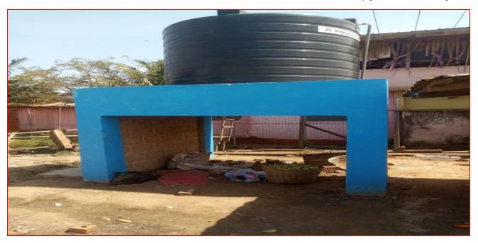
7. Extension and Construction of 3 No. concrete Stands for installation of Rambo 1000 polytank completed at Agona Nkwanta supplying quality water beneficiary
