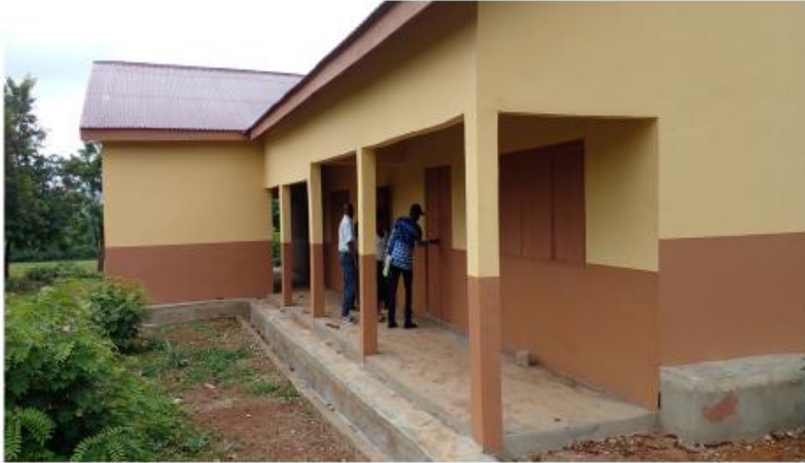
3 Unit classroom block at Sayeraso
