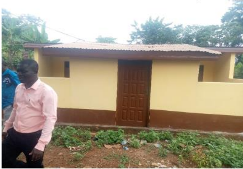
1No. 6 Seater WC toilet at Juaboso Magazine
