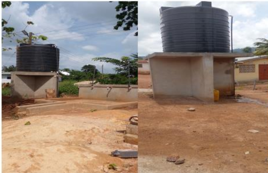
Mechanised boreholes at Dominibo and Boinzan
