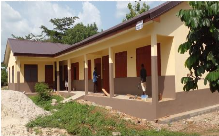
3 Unit classroom block at Danyame
