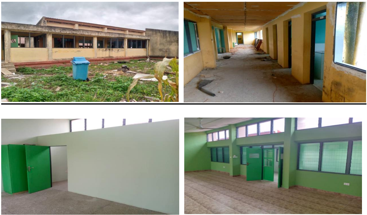
Figure 5: Renovation of Maternity Ward at Kpedze Polyclinic Before And After
