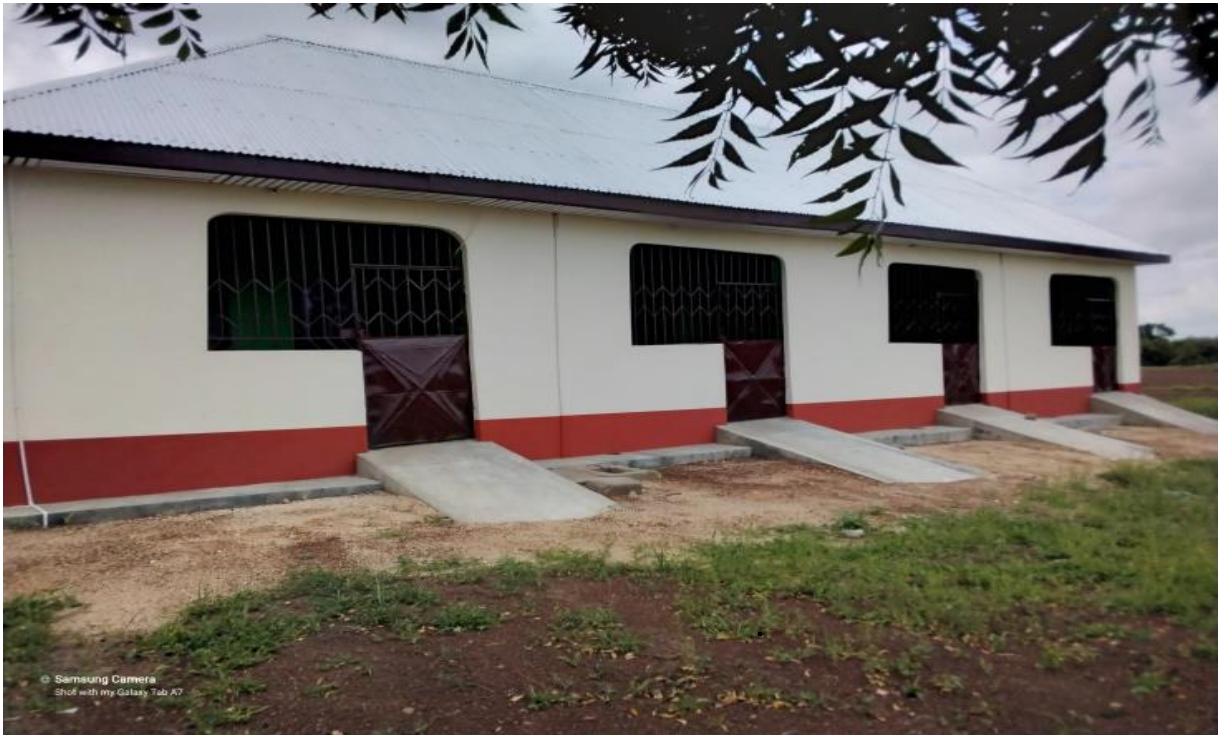
Construction of 2Units 4 No. staff quarters with mechanized borehole at Funsii-DDF
