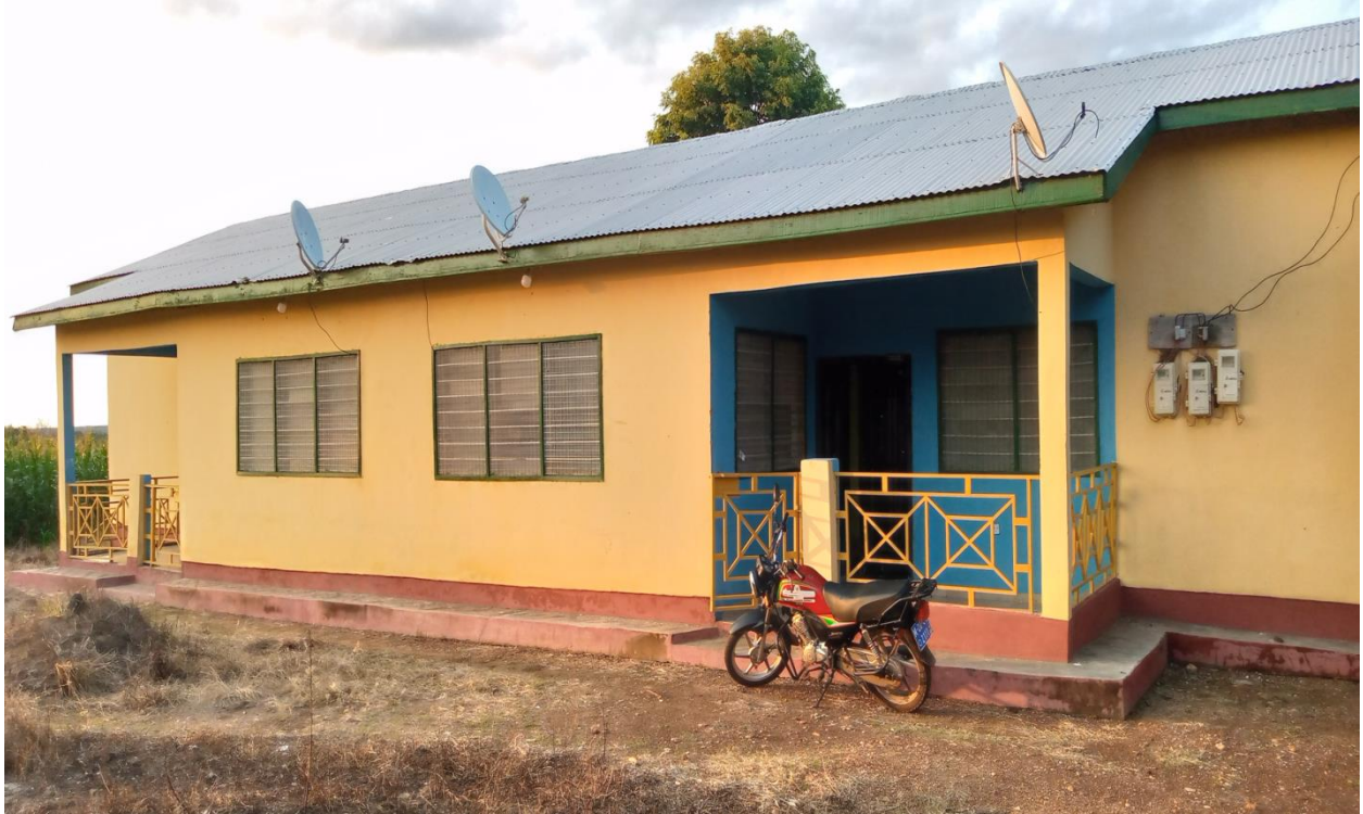
Renovated 1no. 2units semi-detached staff bungalow
