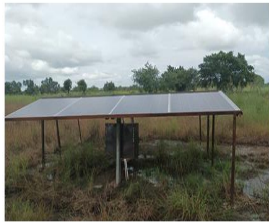
Solar pump irrigation installed at Dabateng for dry season farming (Water Resources Commission)
