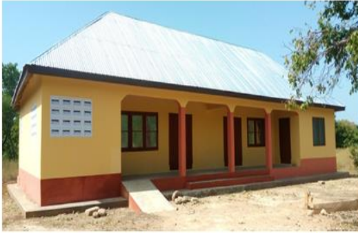
Constructed and Furnished 1no. KG Block at Naapal (MP's Common Fund)
