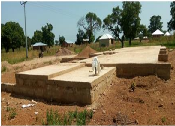
On-going Construction of 1no. CHPS Compound at Vapuo (MP's Common Fund)
