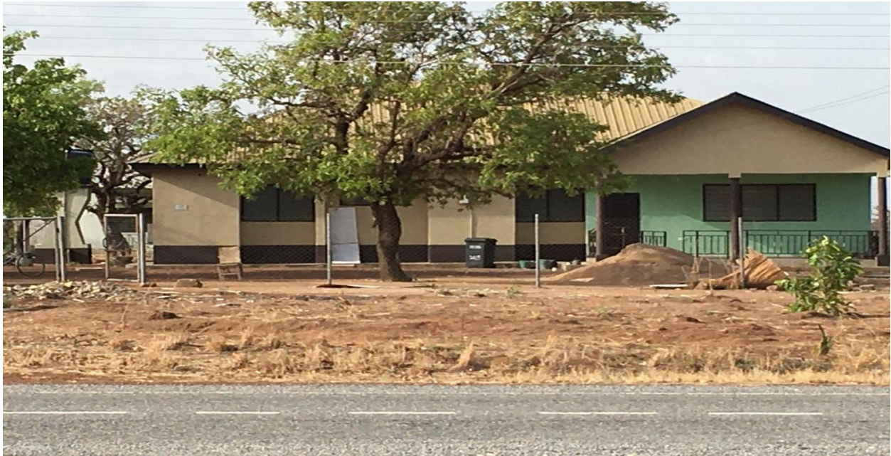
REHABILITATED DA STAFF BUNGALOW AT ISSA
