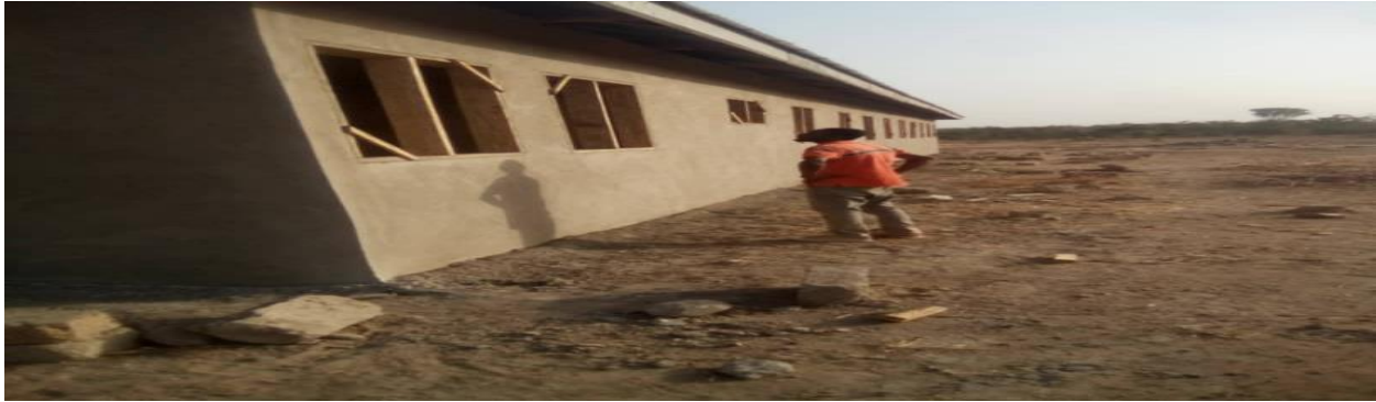
1NO. 3-UNIT JHS CLASSROOM BLOCK UNDER CONSTRUCTION AT DUANG
