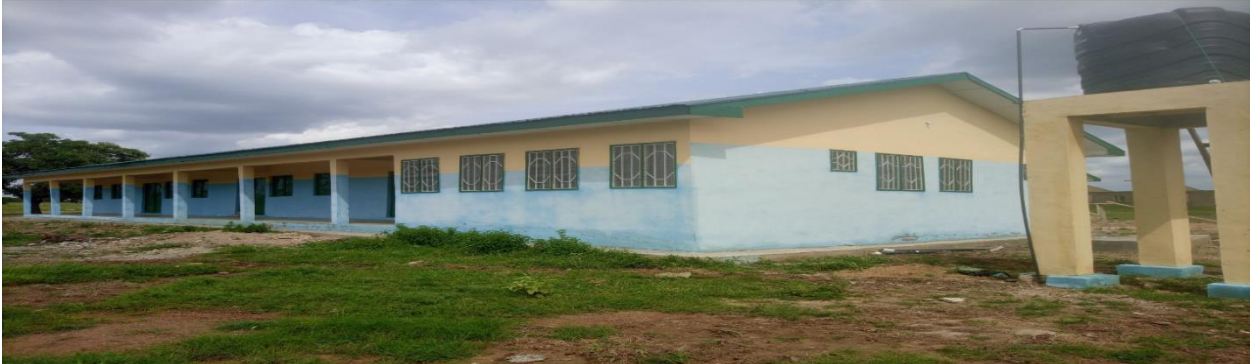
CONSTRUCTED 2NO. 3-UNIT CLASSROOM BLOCKS AT TABIASI
