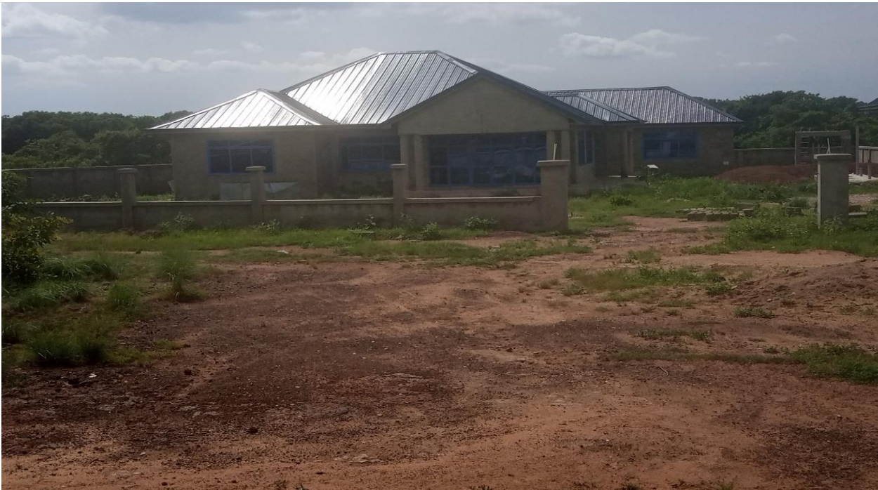
1NO. NHIS OFFICE COMPLEX UNDER CONSTRUCTION IN ISSA
