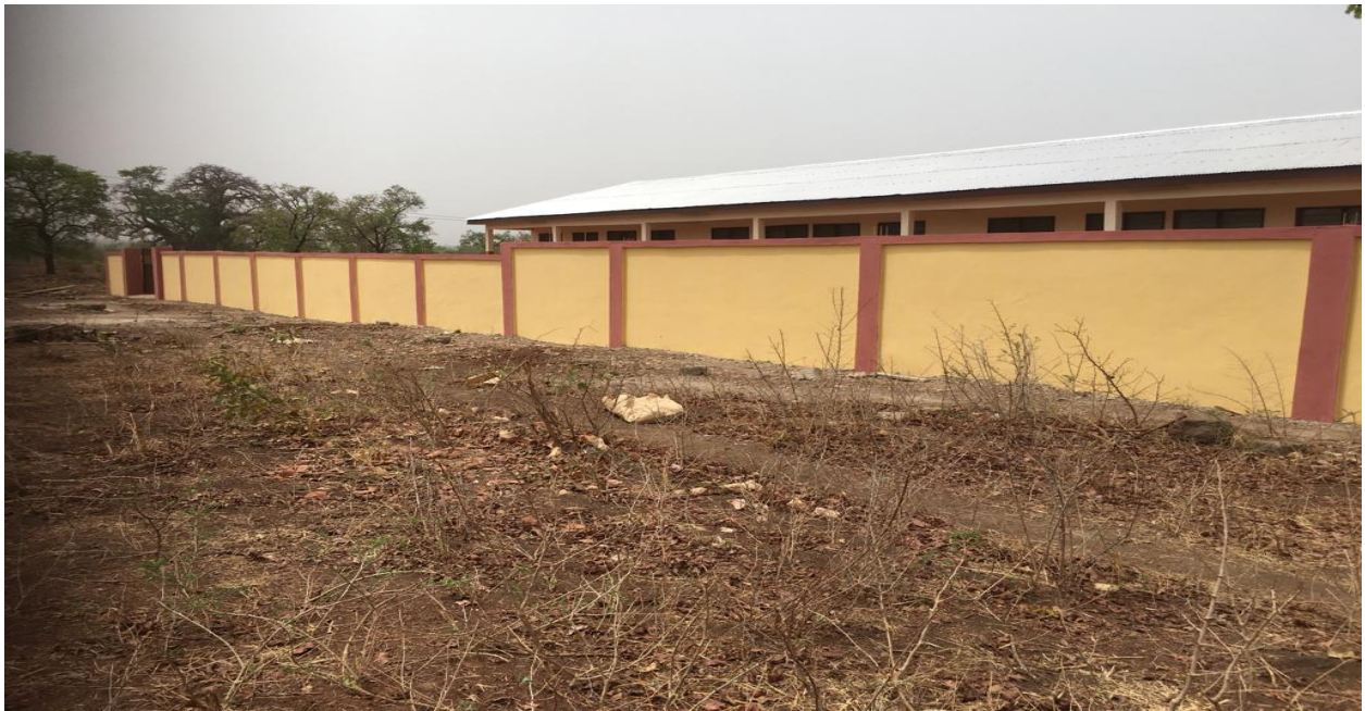
CONSTRUCTED 1NO. FENCE WALL FOR ISSA SHS DORMITORY BLOCK
