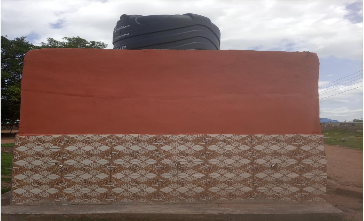
MECHANIZED 1NO. BOREHOLE AT KOJOKPERI MARKET
