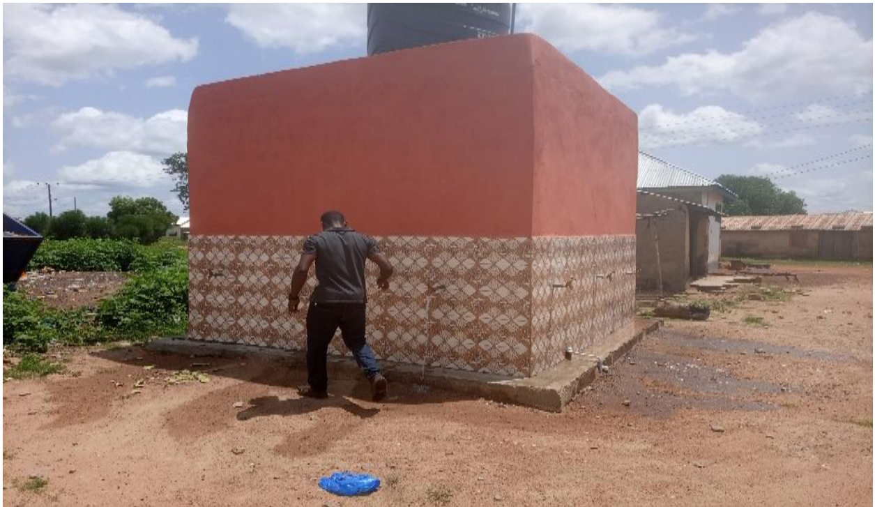
MECHANIZED 1NO BOREHOLE AT DAFFIAMA MARKET
