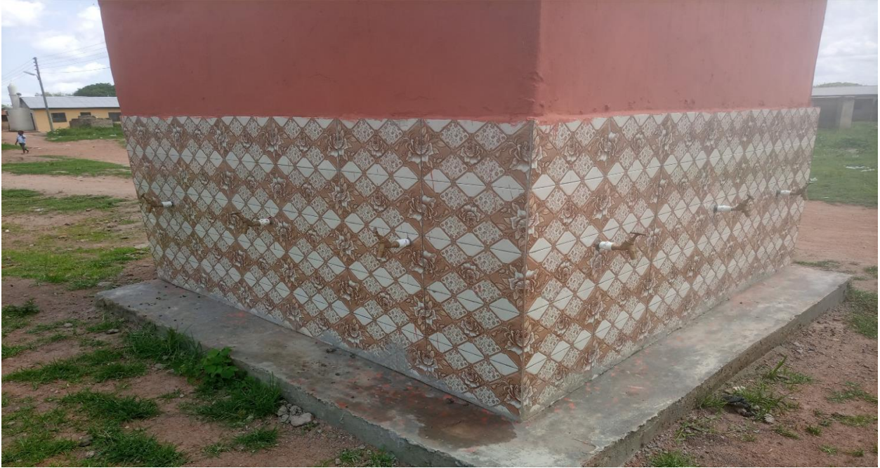
MECHANIZED 1NO. BOREHOLE AT ISSA MARKET
