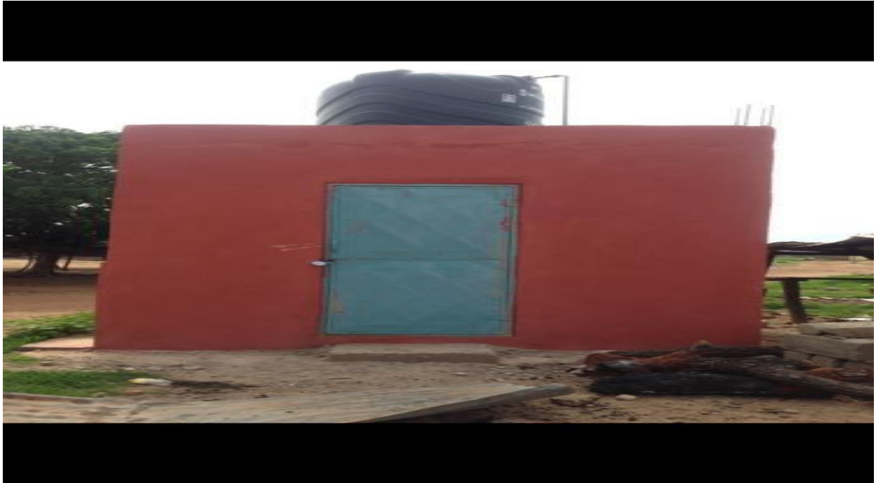
MECHANIZED 1NO. BOREHOLE AT BUSSIE MARKET
