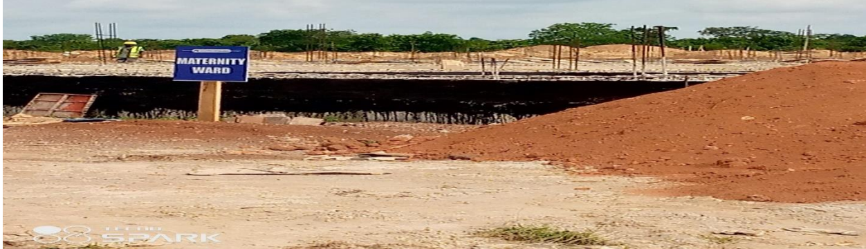
AGENDA 111 DISTRICT HOSPITAL UNDER CONSTRUCTION IN ISSA
